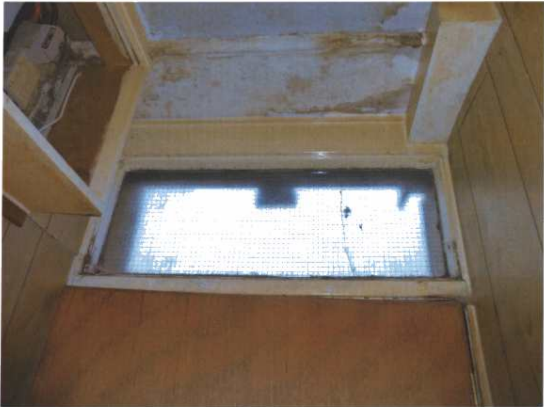
Fanlight above entrance door
