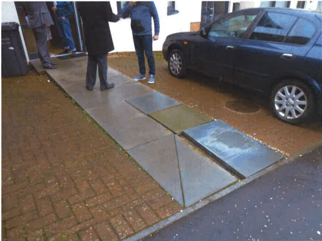
Footpath to front of house
