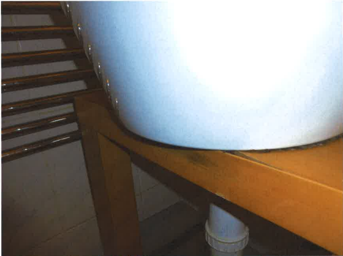
Minor warping of sink stand/ledge
