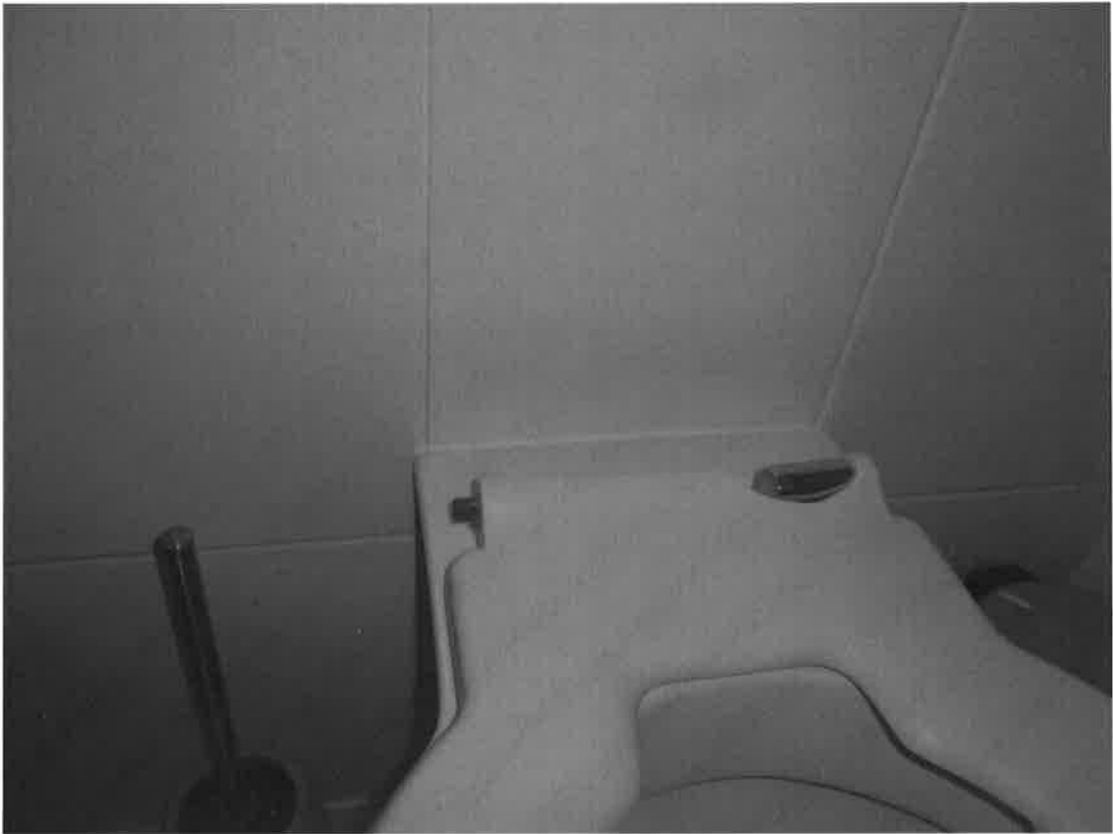
Damaged toilet seat
