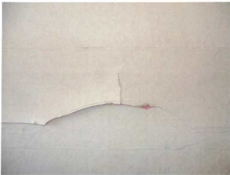
Wallpaper rear left bedroom
