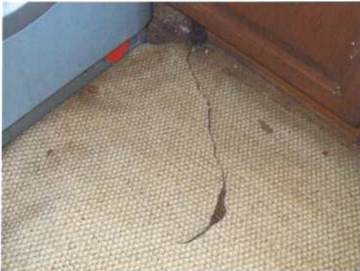
Kitchen vinyl floor covering
