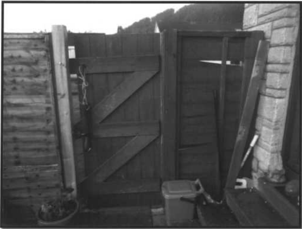
Figure 9 Damaged gate
