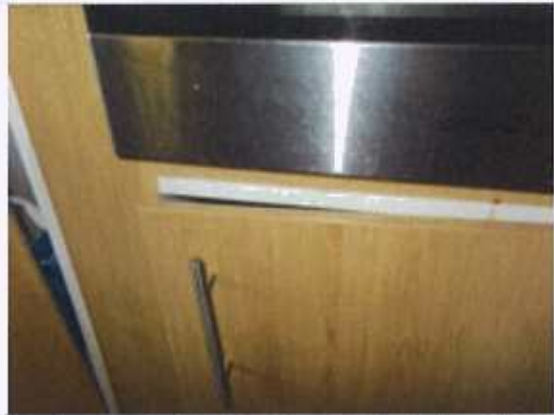
Kitchen cabinet doors
