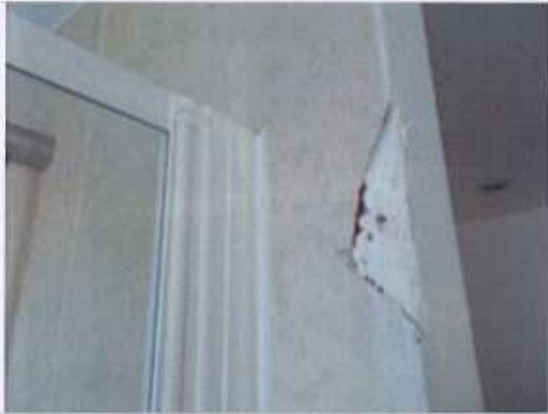
Wall adjacent to shower in bathroom
