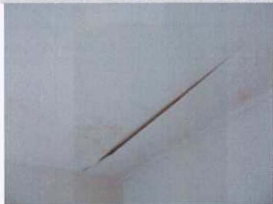
Rear double bedroom ceiling
