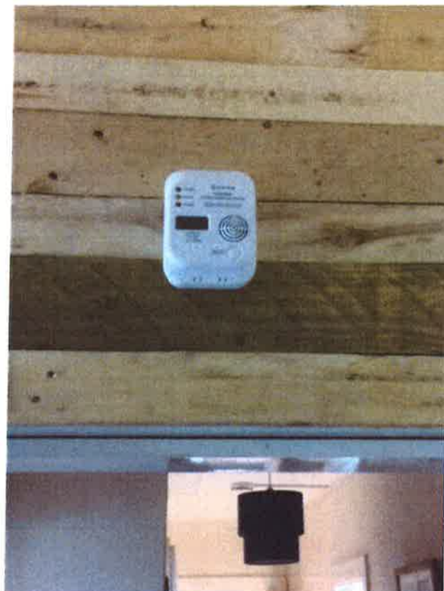
Carbon monoxide detector – kitchen
