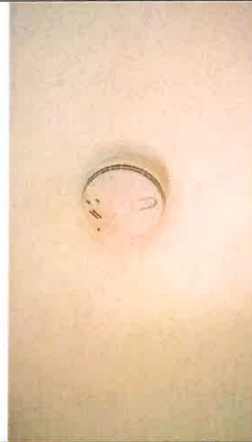
Hard Wired Smoke Detector
