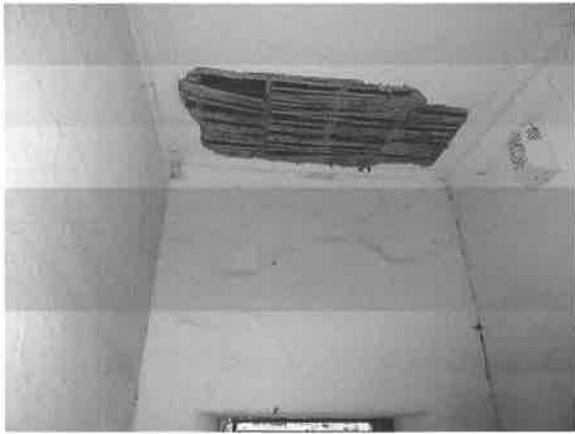
Photograph 4:- Missing, bossed, cracked & damp ceiling plaster at close stairwell.
