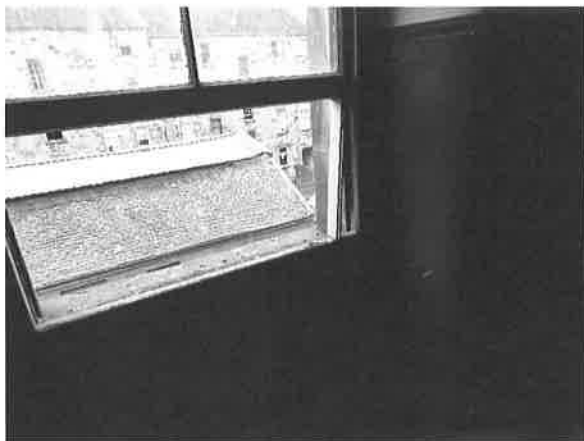
Photograph 5:- Defective sash window jammed open close stairwell
