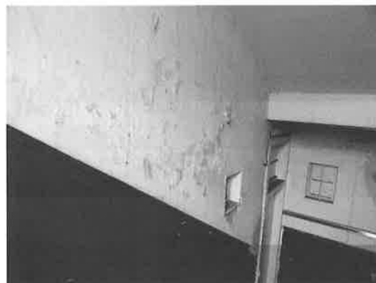
Photograph 5:- Defective sash window jammed open close stairwell
