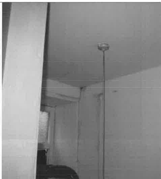
Water penetration common close wall
