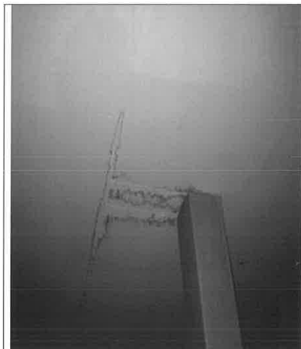
Water penetration common close ceiling
