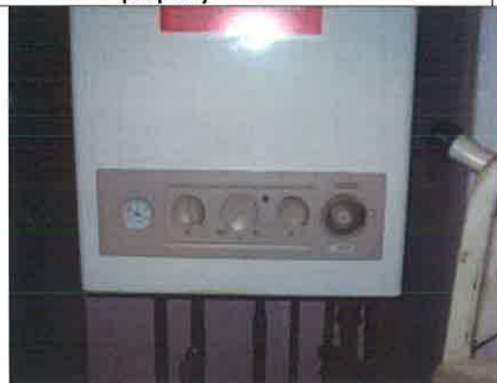
Gas boiler ( no CO Monitor )
