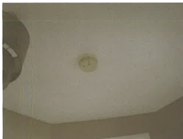
Smoke detector-upper landing
