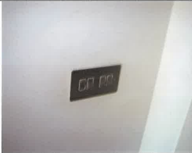
Photo 5 – Booster switch (left) for fan
