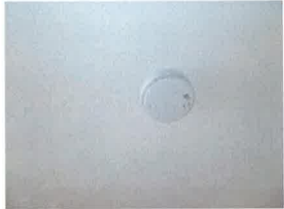
Living Room - ceiling mounted smoke alarm
