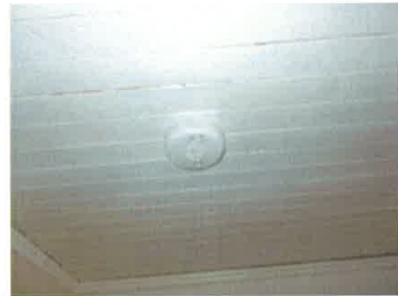
Kitchen - ceiling mounted heat alarm
