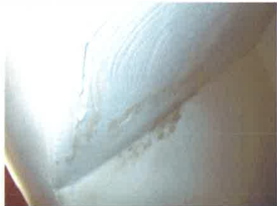
Living Room - damp patch to camceil ceiling/wall on right side of dormer window
