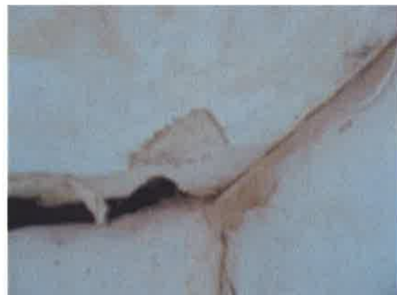
Back Bedroom - camceil ceiling to right side of dormer window showing closer view of water damage to plasterboard
