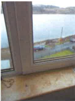
Front Bedroom window - showing water staining to sill
