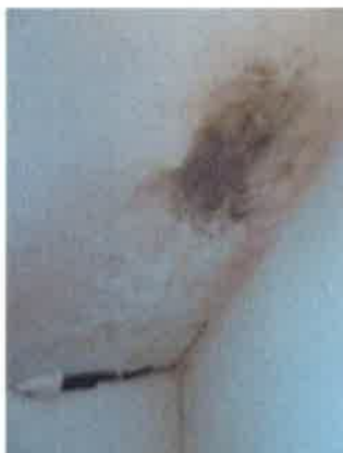
Back Bedroom - camceil ceiling to right side of dormer window showing water damage to plasterboard and black spot mould
