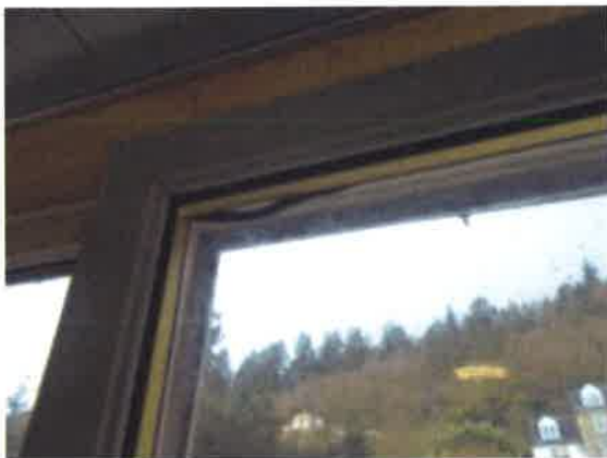
Kitchen window - showing dislodged seal
