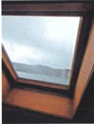
Box Room - Failed seal to Velux window - condensation between double glazing panes
