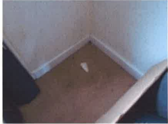
Back Bedroom - water stain to carpet under camceil ceiling on right side of dormer window
