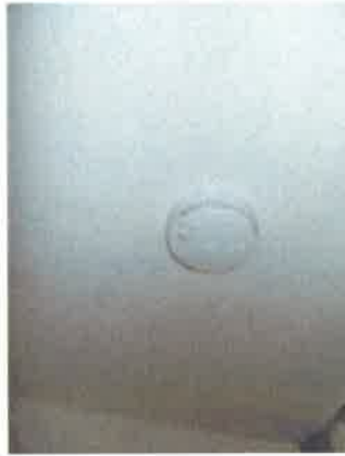
Hall - ceiling mounted smoke alarm
