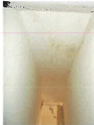
Internal staircase - damp patch to ceiling
