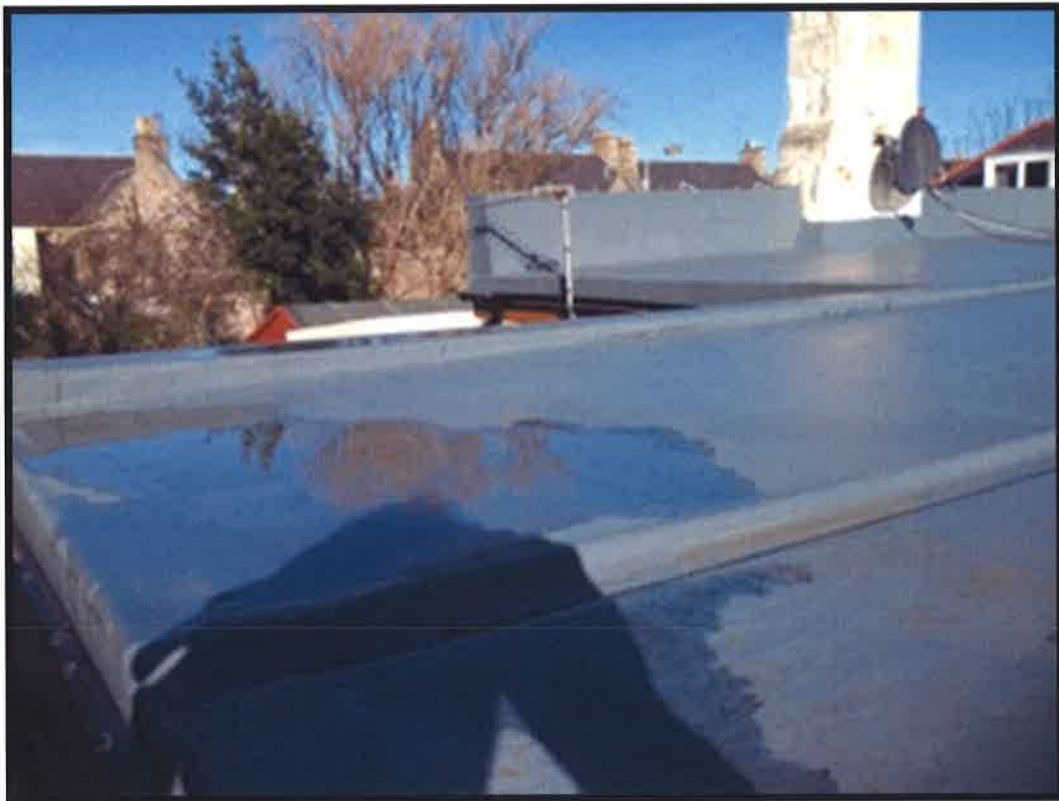
Figure 22 Rear section of flat roof with ponding over bathroom.
