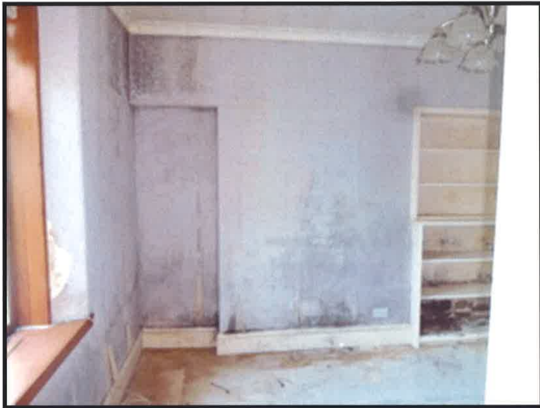
Figure 10 Rear bedroom -extensive mould and damaged wallpaper.
