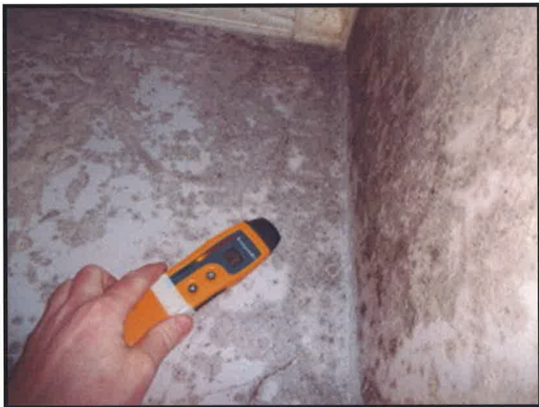
Figure 8 Rear bedroom - Meter reading (16%) high level rear corner and heavy mould growth.
