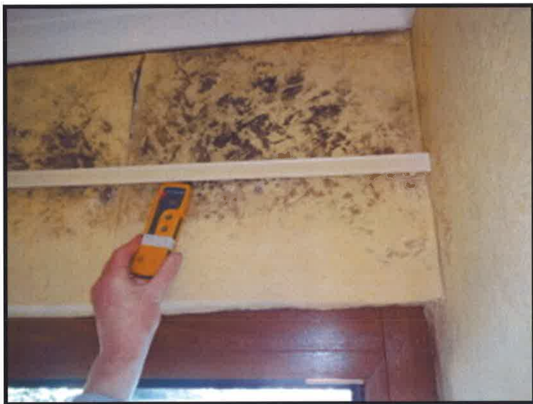
Figure 20 Rear hall - moisture meter reading (100%)
