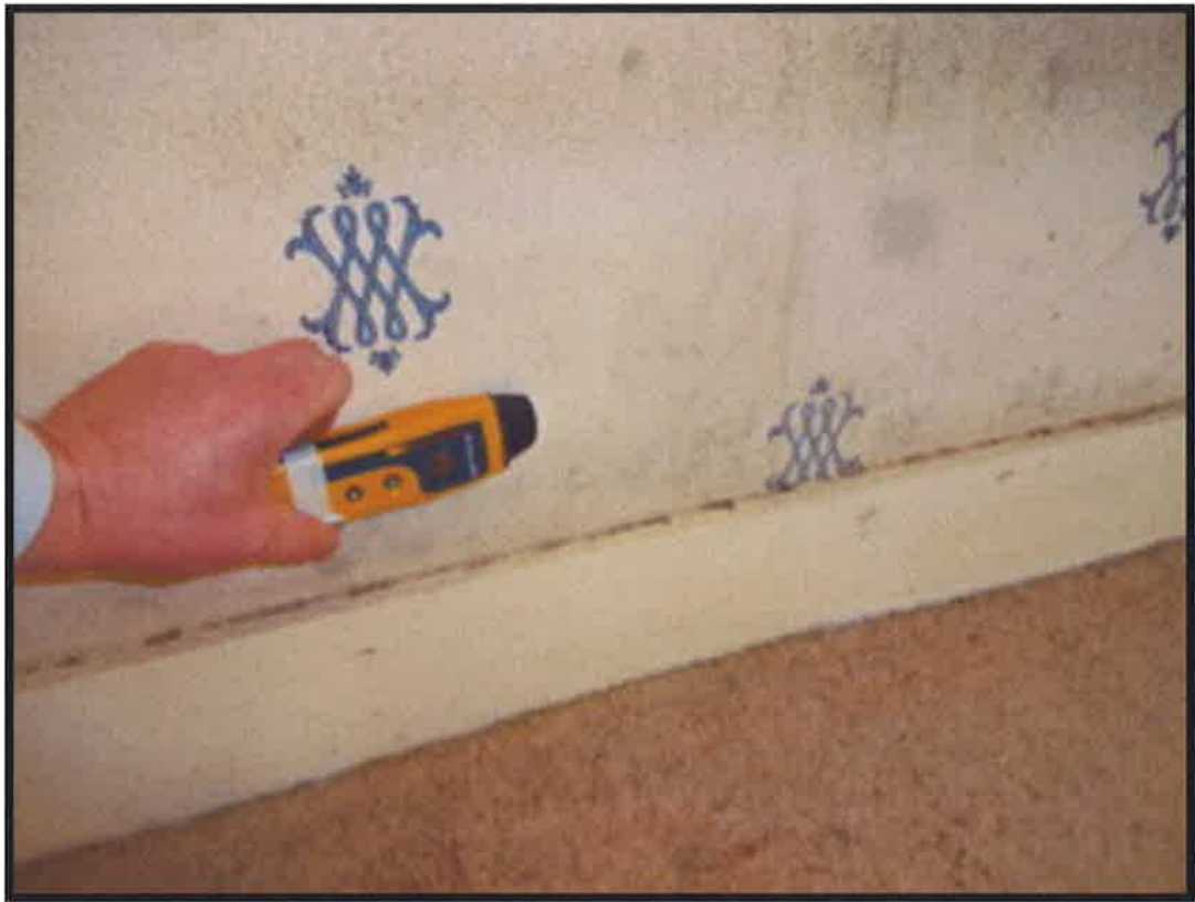
Figure 8 Middle Bedroom - Meter reading (18%) and soiled decorations
