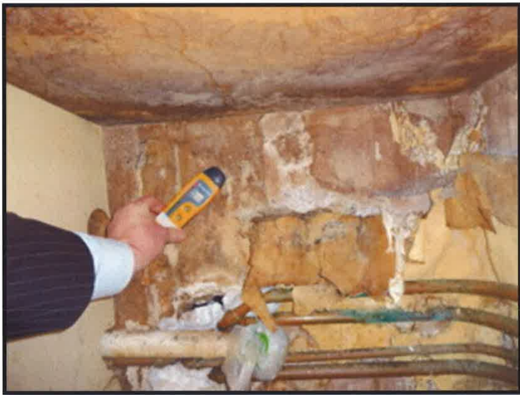
Figure 126 Kitchen - rear wall at site of dishwasher moisture meter reading (100%)
