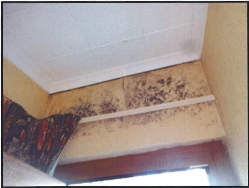
Figure 159 Rear hall - mould above rear entrance door.
