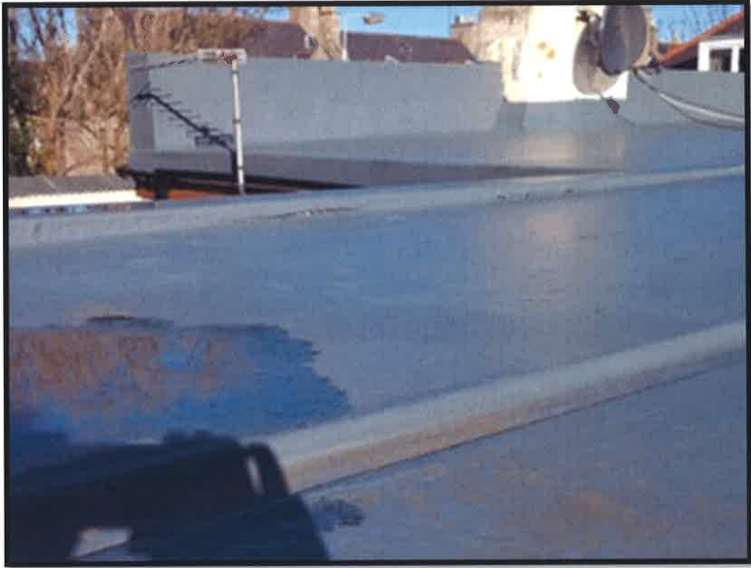
Figure 23 Rear section of flat roof with gap above rear entrance door.
