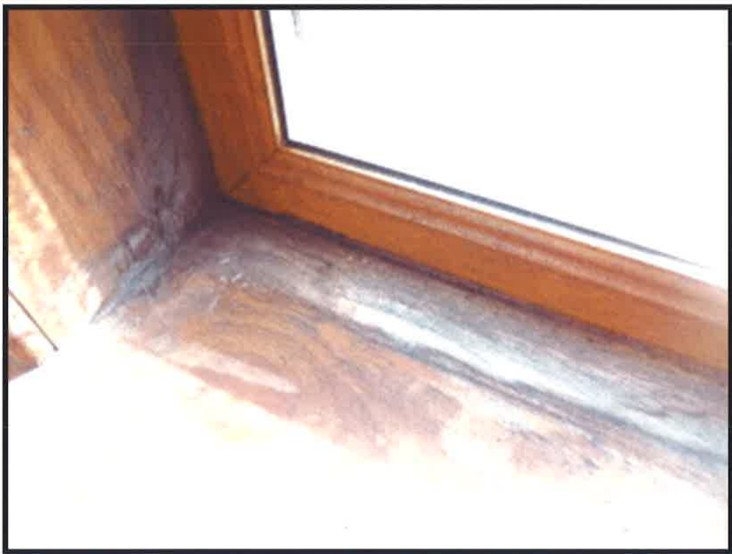
Figure 9- Middle bedroom - water marks to timber window cill.
