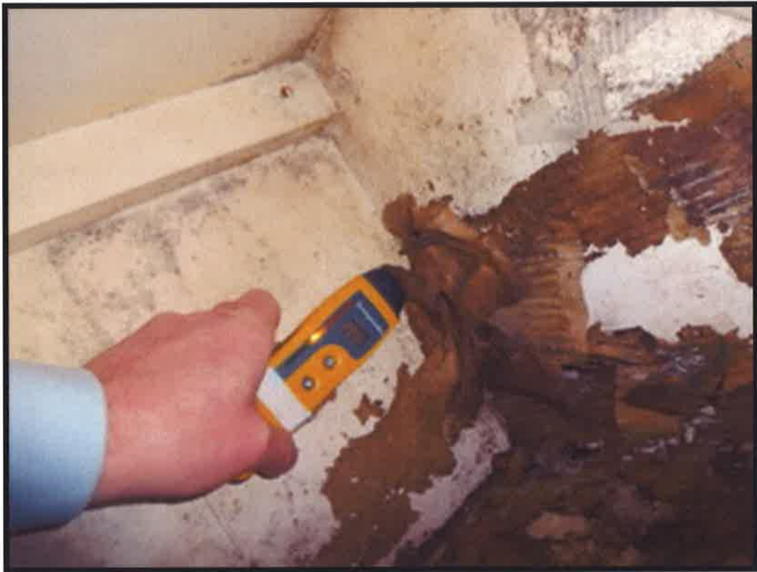
Figure 7 Rear bedroom - Meter reading (19%) within alcove and residue of cardboard box.
