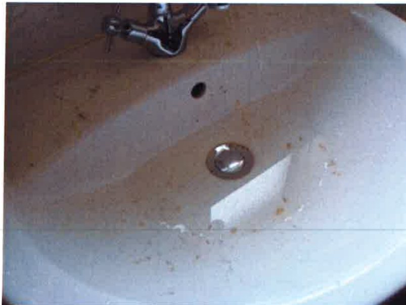
DEFECTIVE MECHANISM AT PLUG
