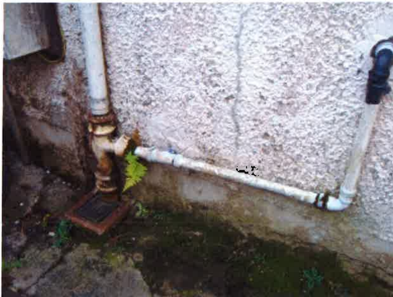
EXTERNAL DRAINAGE PIPE FROM BATHROOM
