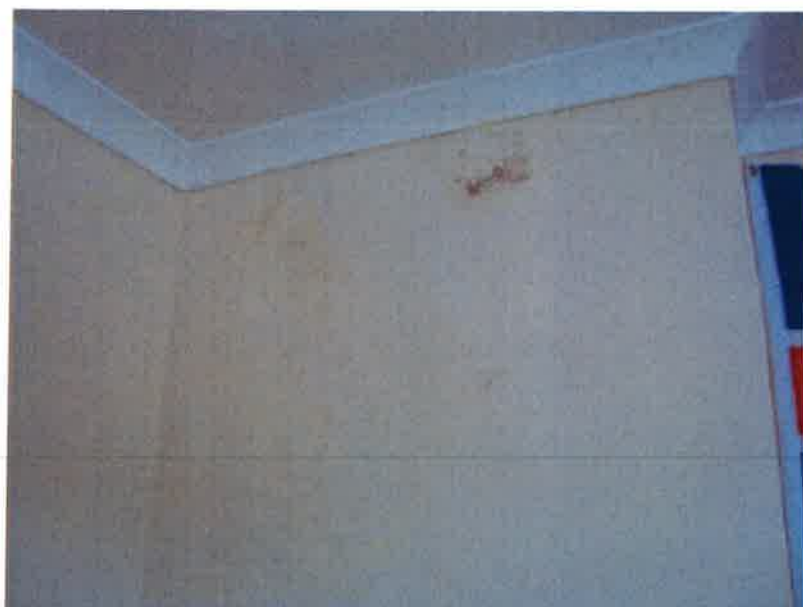
STAINING AT FRONT BEDROOM CHIMNEYBREAST (12/04/17)
