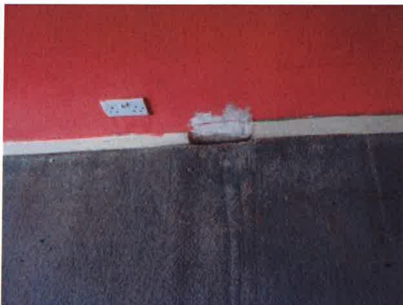
SECTION OF MISSING SKIRTING BOARD (BED 2 ND LEFT)
