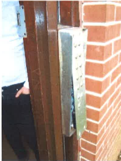
Vandalised door entry panel (Rear door)
