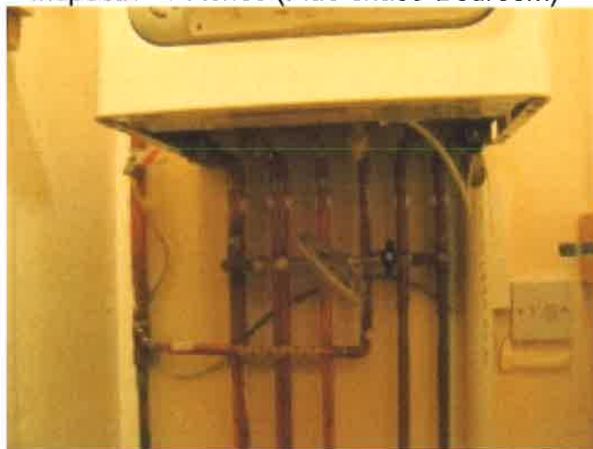
Earth bonding at central heating boiler.
