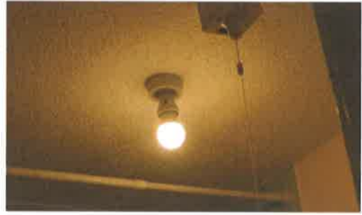
Photo 9 – Bathroom light fitting
