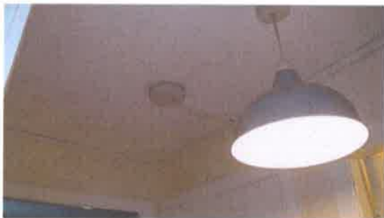
Photo 6 – Smoke alarm in Hallway
