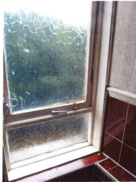
7. Bathroom window showing failed draught stripping
