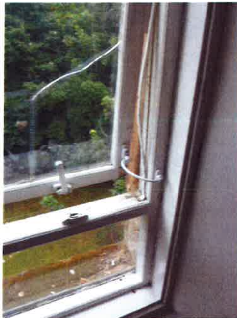
6. Back bedroom window showing failed draught stripping
