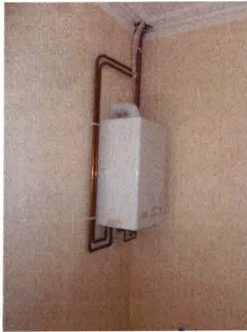
9. Central heating boiler in front bedroom
