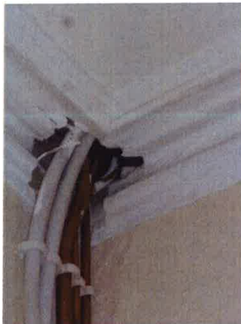
10. Hole in ceiling above boiler
