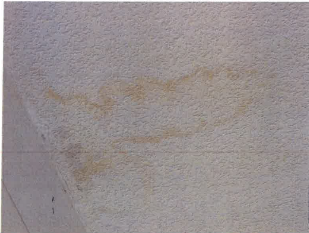
15. Damp staining on Shower Room ceiling
