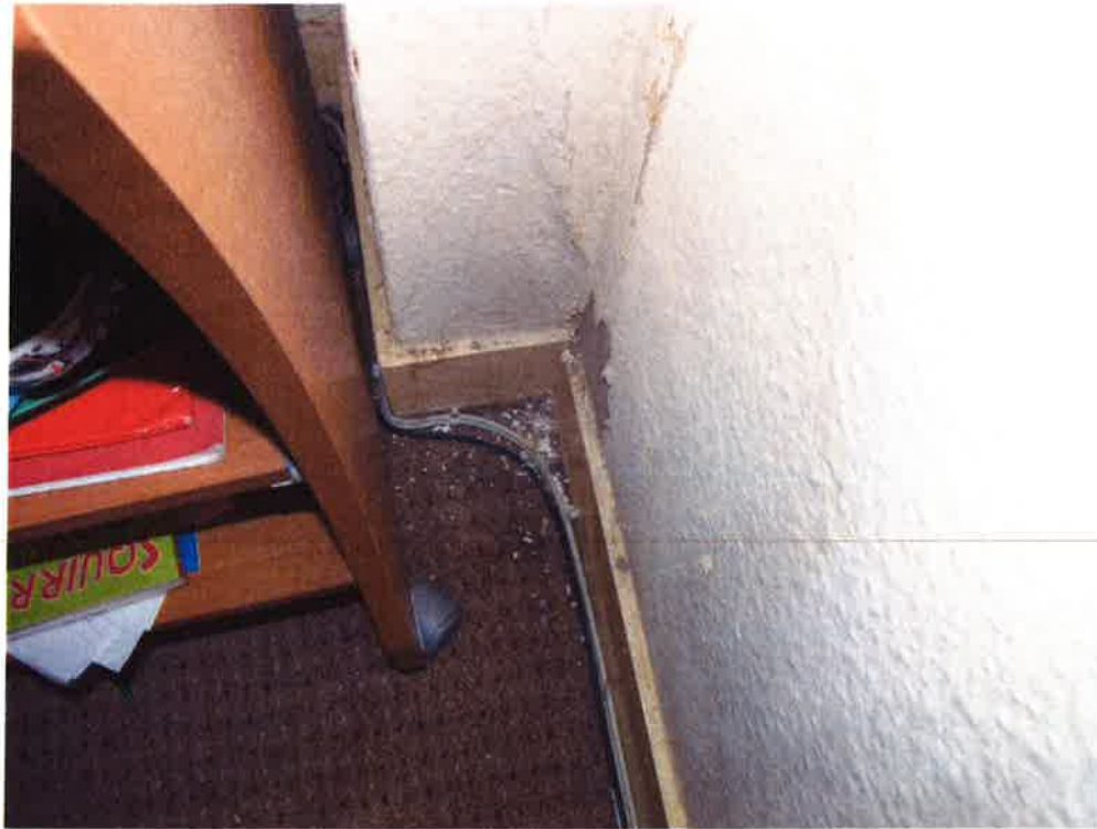
17. Damp staining in corner of rear Bedroom (north)
