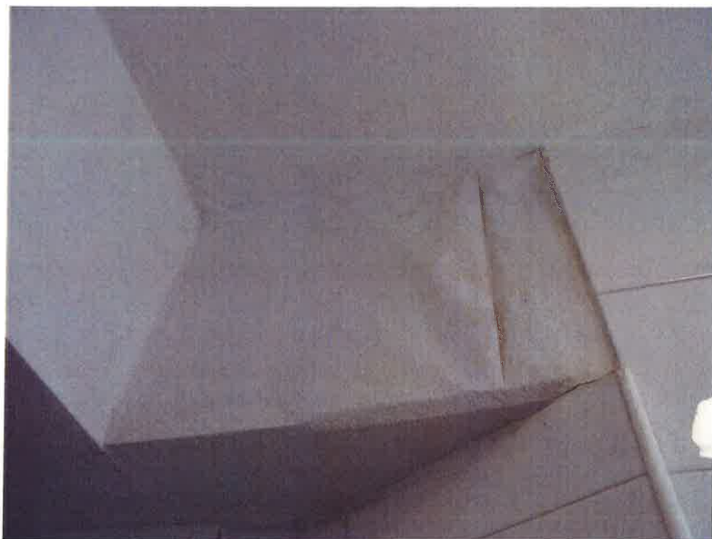
16. Damp staining on Shower Room upper wall
