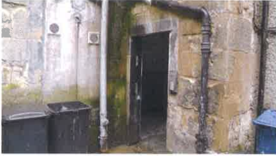
Photo 2 – Ground floor access at rear + side
