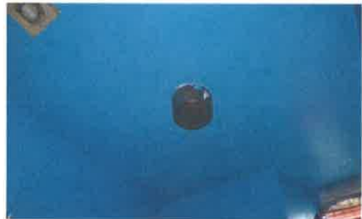
Photo 5 – Ceiling light fitting in bathroom
