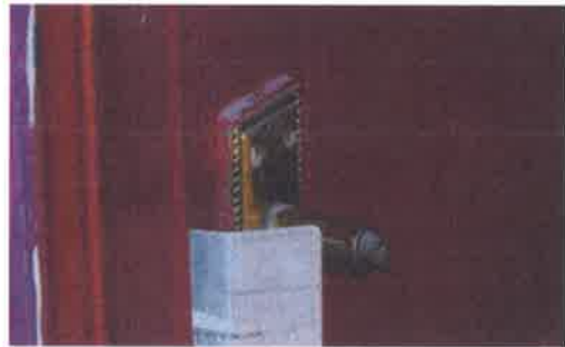
Photo 13 – Door handle into boiler cupboard
