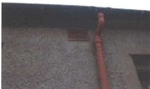
VENT - FRONT WALL
