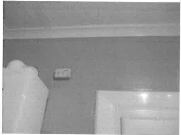
Kitchen - wall mounted Carbon Monoxide alarm situated just above and to the right of the boiler
