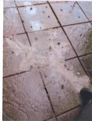
Rear paving stones - cracks repaired with mortar
