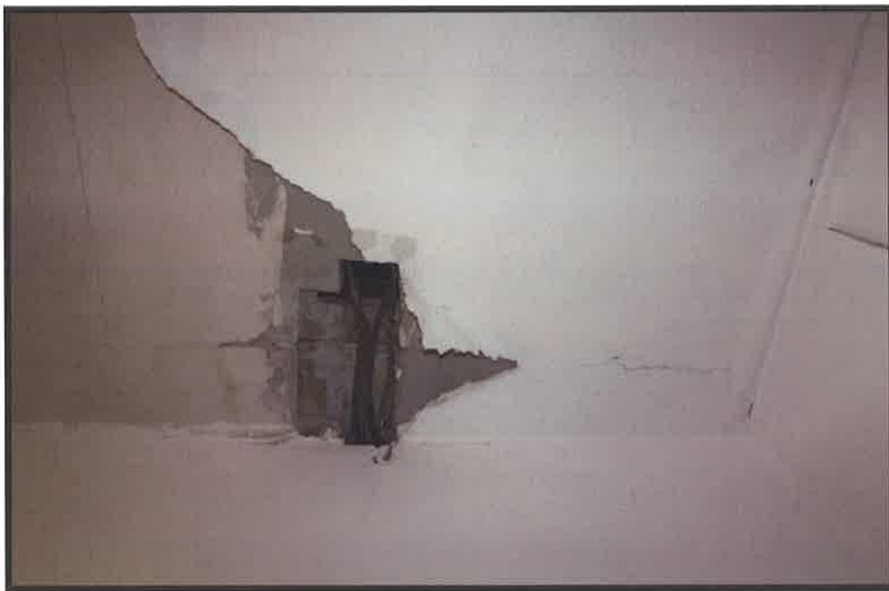
Figure 6 Inner hall ceiling
