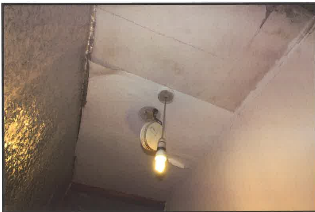
Figure 7- Inner hall ceiling - smoke alarm.
