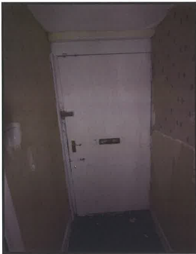
Figure 2 Inside face of front door.
