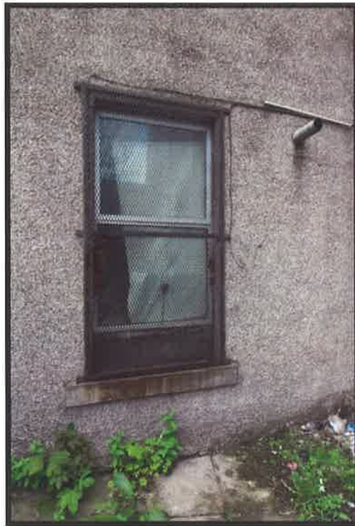
Figure 16 Rear window and bathroom vent.
