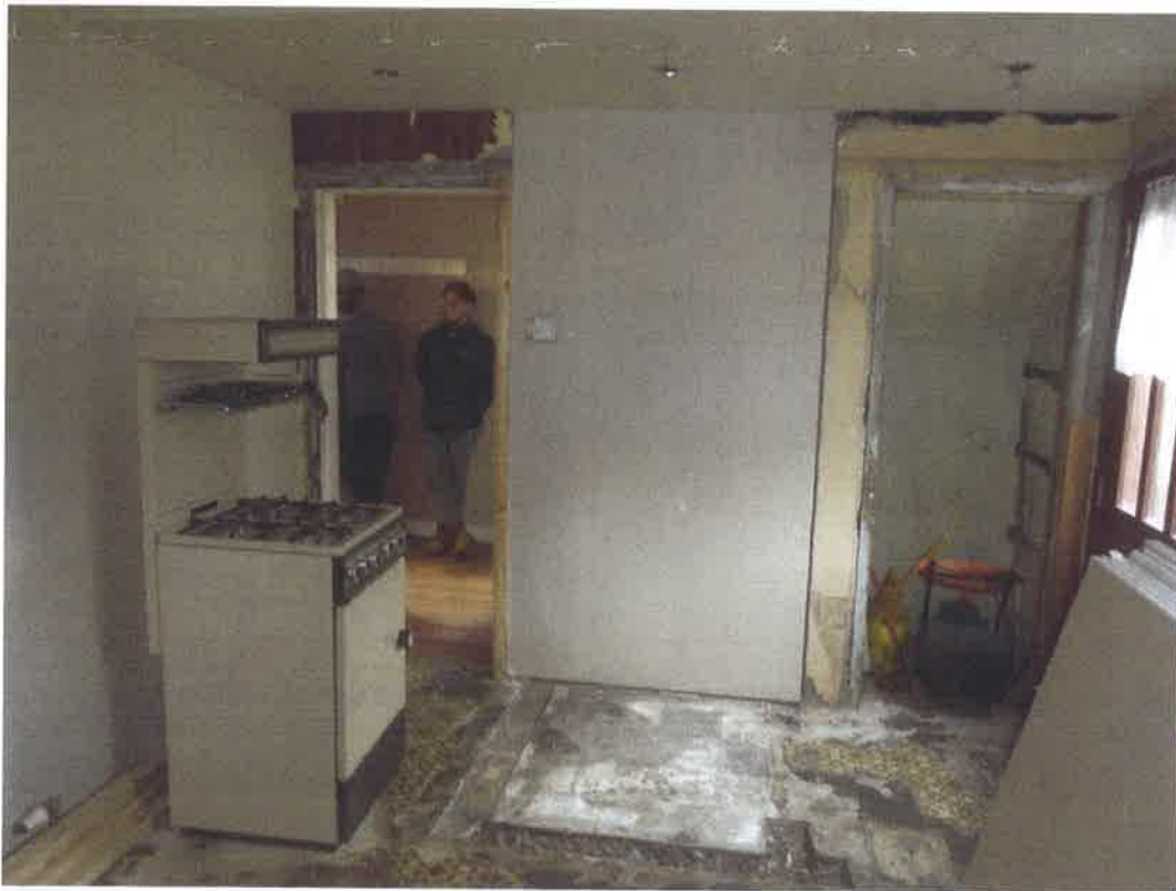
Kitchen – showing where walls taken down and wall linings removed
