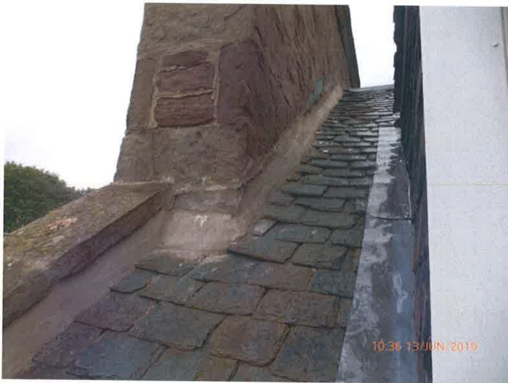
Recent repair to flashing
