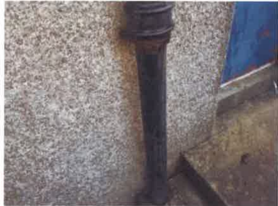
32 Cast iron downpipe.
