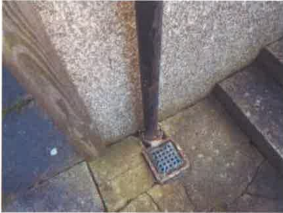
31 Cast iron downpipe.
