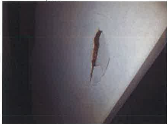
16 Further example of damage to pass door.
