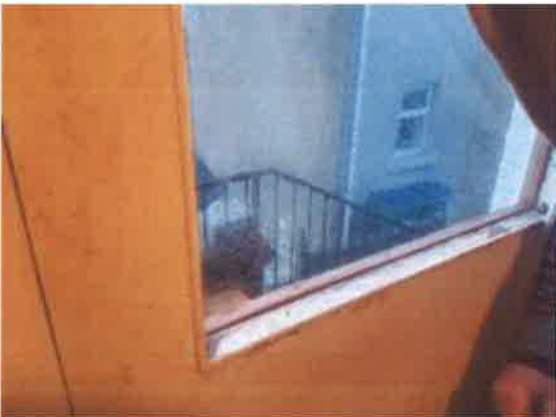
3 Rear entrance door.
