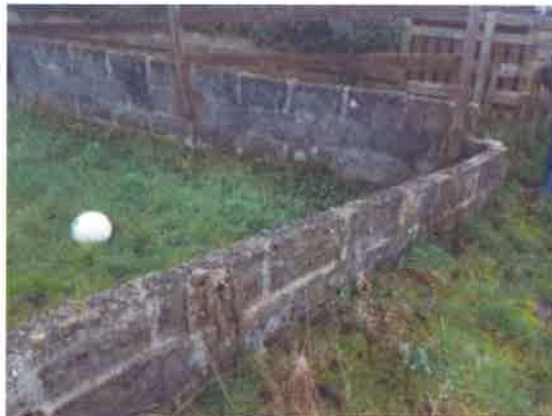
44 Blockwork boundary wall.
