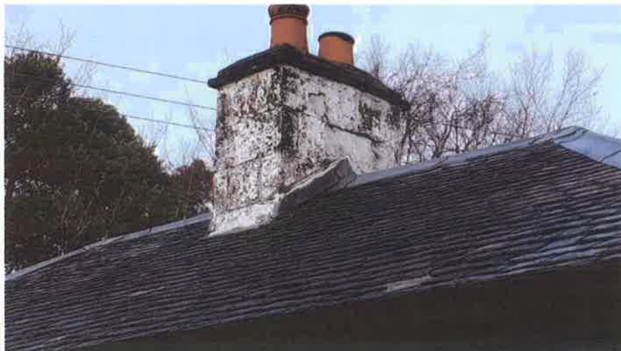
2 The front chimney (stonework, pointing and pot haunching defective)
