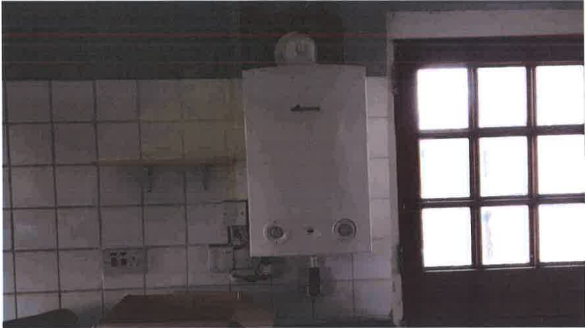
15 The kitchen boiler (no CO detector)
