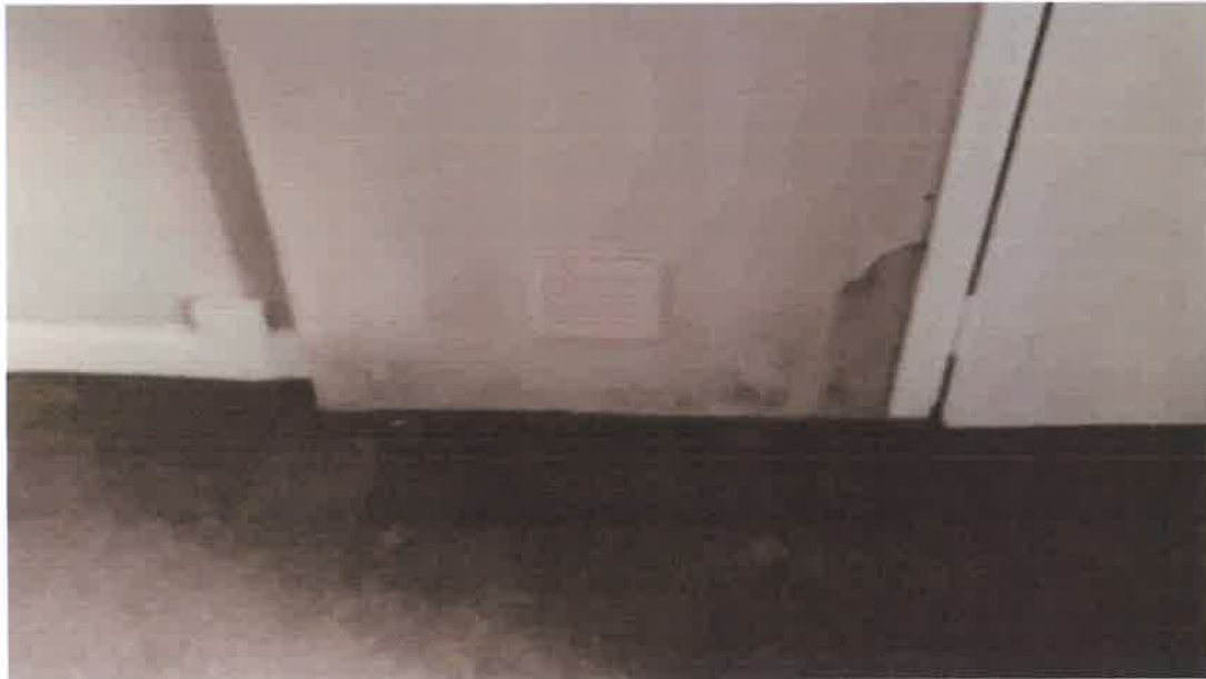
11 Dampness at rear chimney breast in bedroom 2
