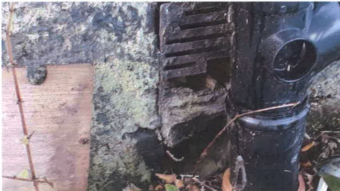
8 The side elevation east (hole in stonework and defective air vent)
