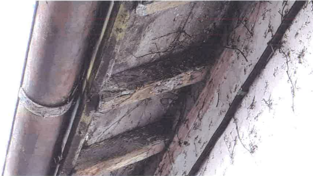
7 An example of a defective section of the timber soffit at eaves
