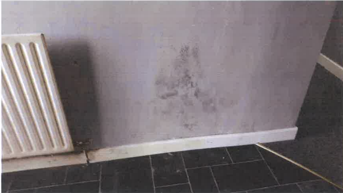
9 Dampness in kitchen wall (separating wall from rear bedroom 2)
