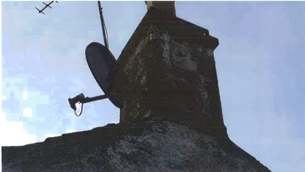
3 The rear chimney (stonework and pointing defective)
