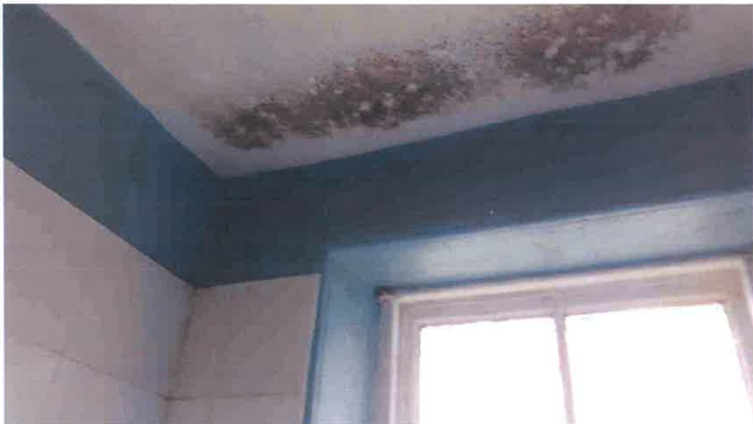
14 Dampness on ceiling in bathroom
