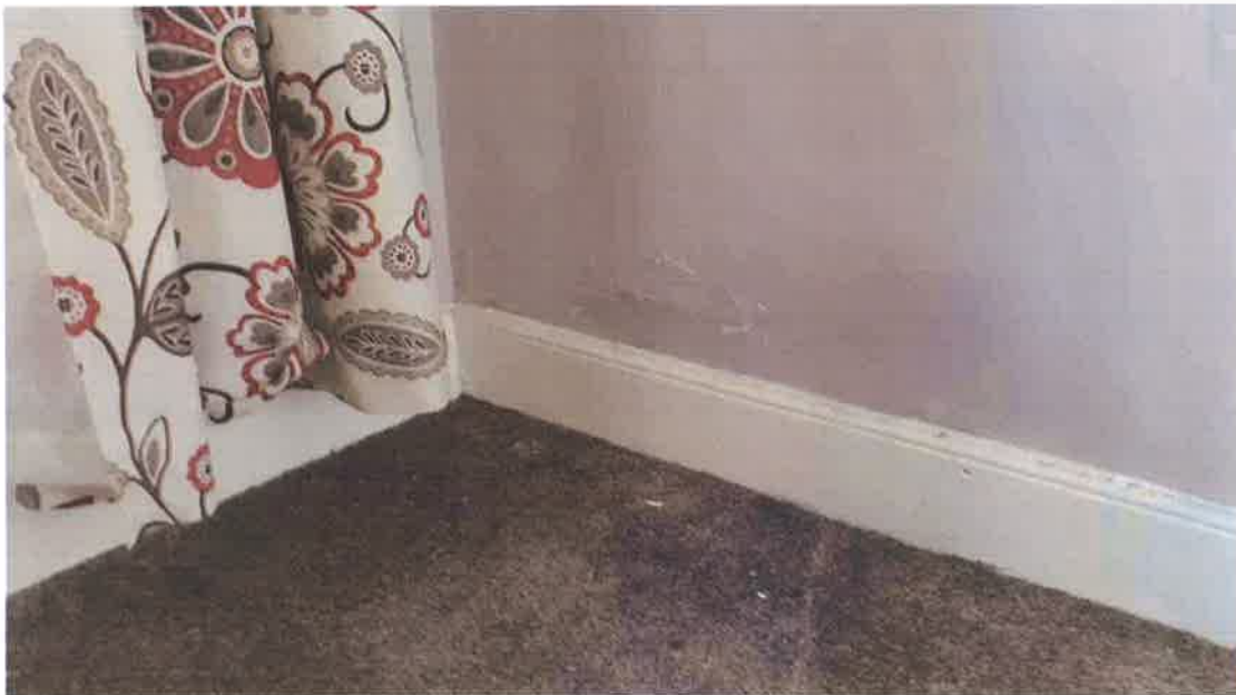
12 Dampness at south east corner at base of wall in bedroom 2
