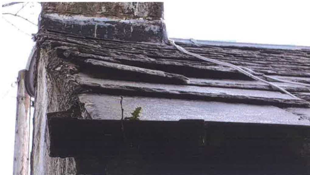
4 The rear roof gable end (defective cement mortar pointing)
