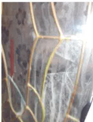
Hall - Front Door - glass broken to decorative glazed panel
