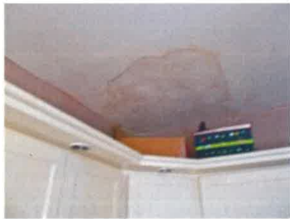
Kitchen Ceiling - large patch of damaged plaster, incomplete repair
