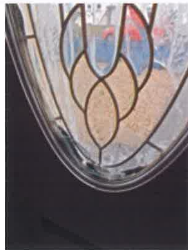
Hall - Front Door - glass broken to decorative glazed panel
