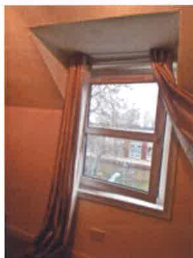
Rear Bedroom (1) Window - defective mechanisms - does not open/close properly
