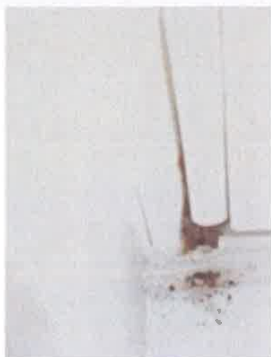
Rear Bedroom (1) Window - hinge corroded
