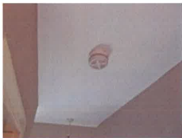
Upper floor landing - ceiling mounted smoke alarm
