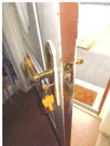
Hall - Front Door - lock sometimes sticks/ possible defect (observation)
