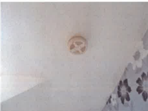
Ground Floor Hall - ceiling mounted smoke alarm
