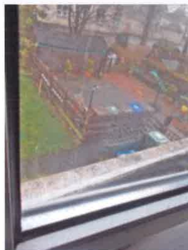
Rear Bedroom (1) Window - double glazing seal broken - condensation between panes
