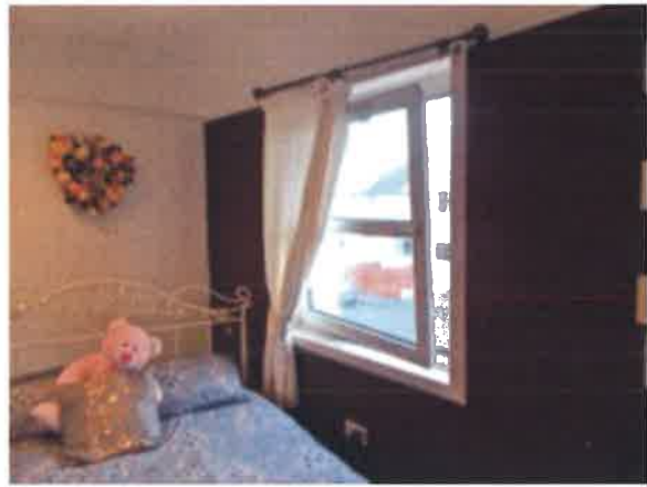
Front Bedroom (3) Left side Window -defective mechanisms - does not open/close properly
