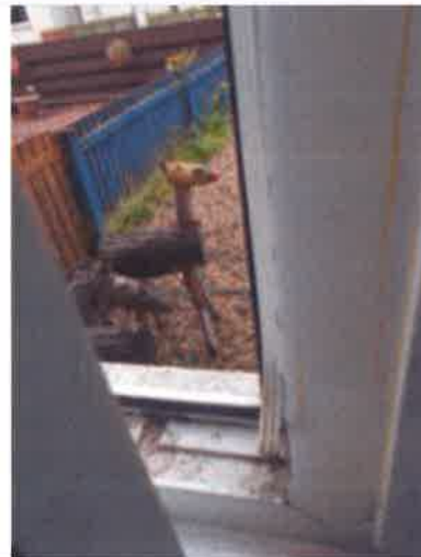
Living Room - left side window seal defective
