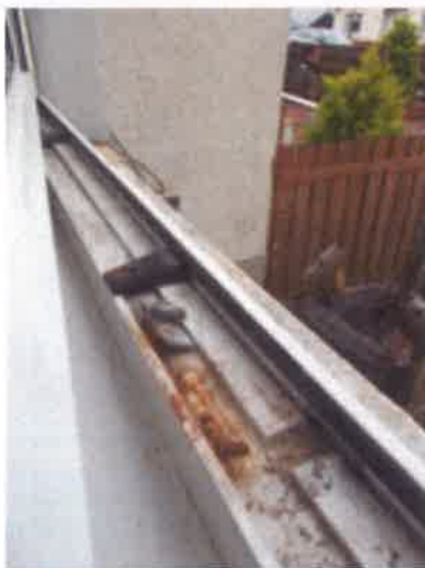
Living Room - Left side window corrosion and defects to mechanisms, does not open/close properly
