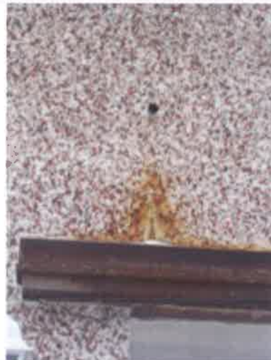
External - water has been running from overflow - roughcast stained and damaged above canopy over front door
