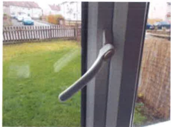
Living Room - main window to left - handle defective/jams when opening/closing
