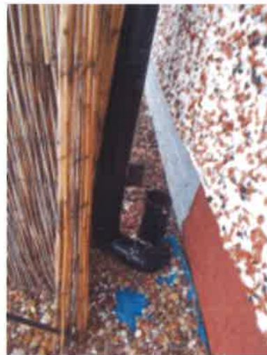
Front elevation - downpipe sections disconnected at base
