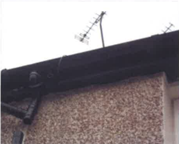
Rear gutter leaking at joints, choked with vegetation
