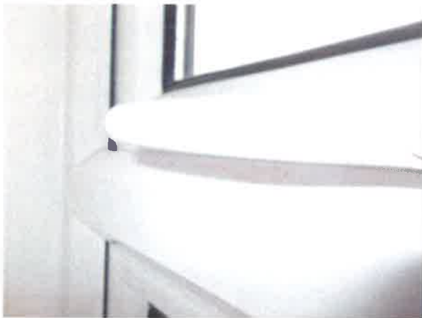
Living Room - top light window to left side does not close properly - gap at seal
