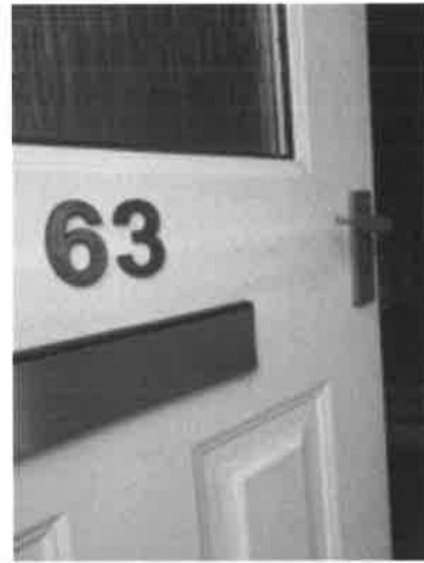
Front Door - no key for mortice lock, cracks to PVC outer face of door
