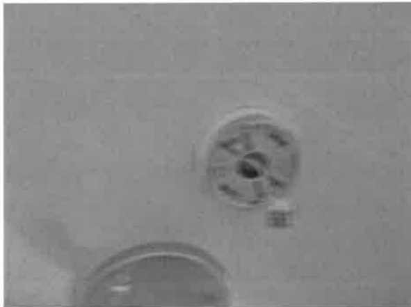
Ground Floor Hall - ceiling mounted smoke alarm - missing cover/exposed wires
