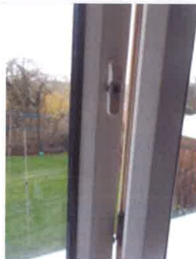
Kitchen - left side window - handle missing
