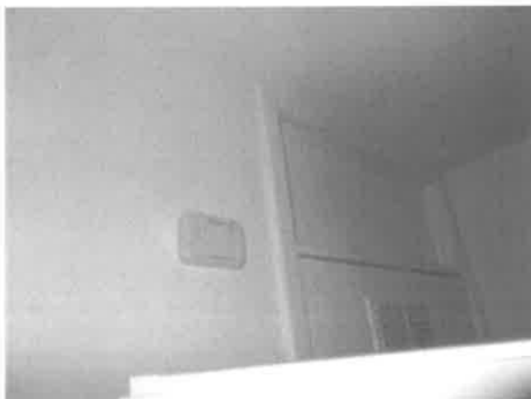
Front Bedroom (1) - Carbon Monoxide alarm - wall mounted, level with top of door to cupboard housing boiler
