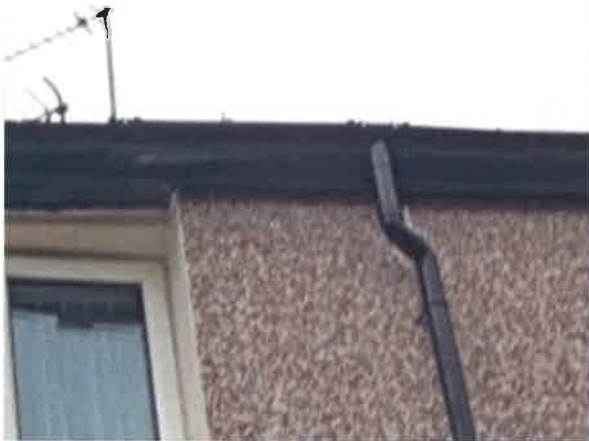
Rear gutter leaking at joints, choked with vegetation
