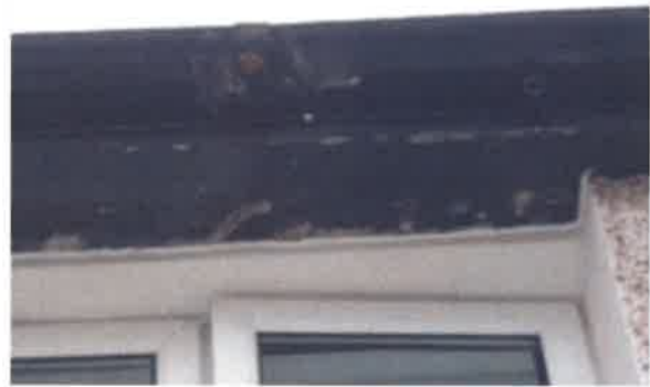
Front gutter leaking at joints and corroded
