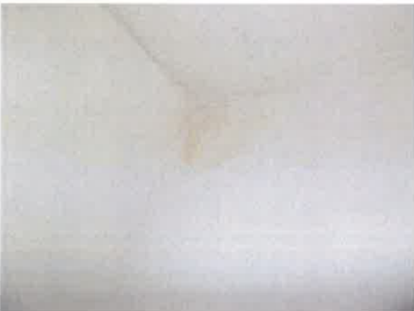
Front Bedroom (1) - staining to front corner of party wall
