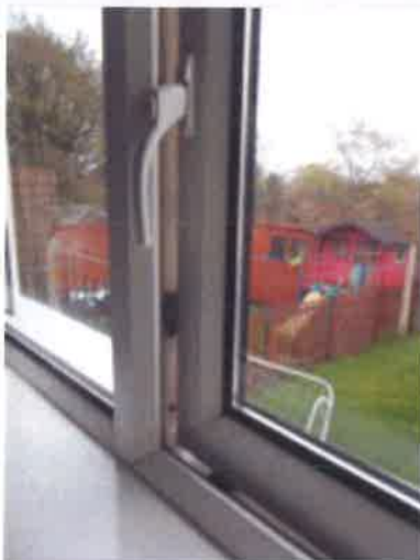
Kitchen - right side window does not close, mechanisms and handle defective
