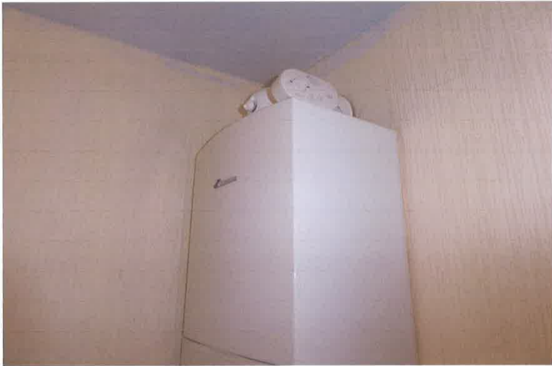
Boiler with carbon monoxide alarm (loose) above.
