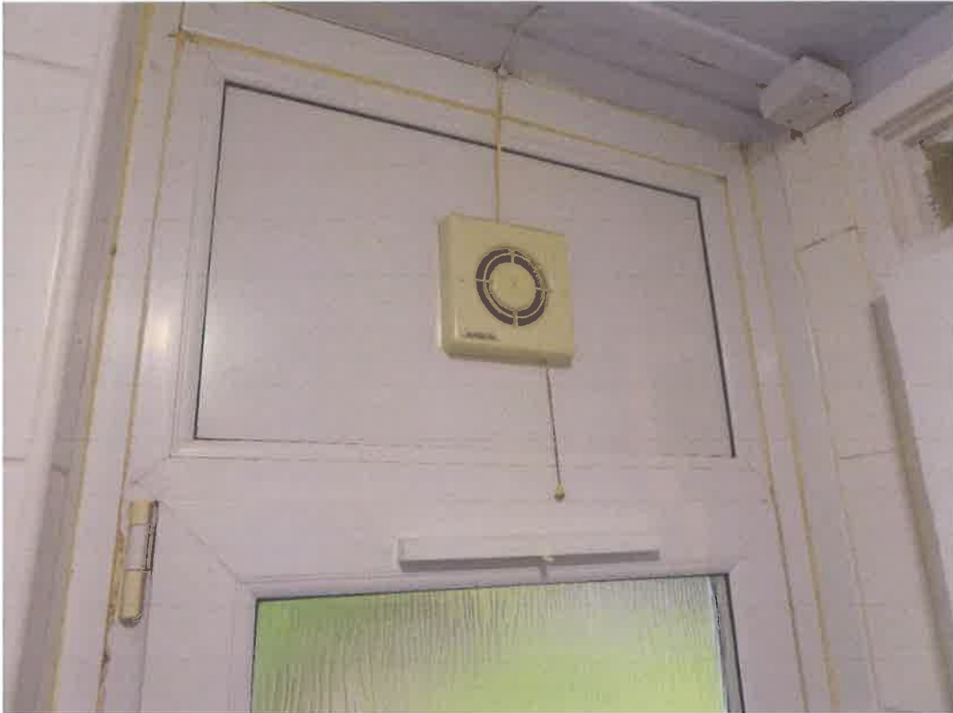
Exelair unit above window with pull switch. Should come on / off with light or humidistat
