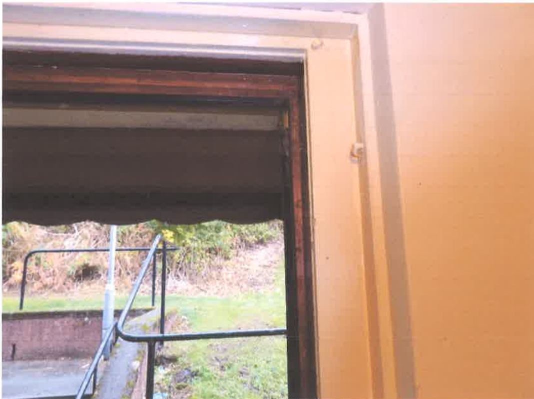
Ground floor Front door seal to door damaged at top section of open side – to be replaced.
