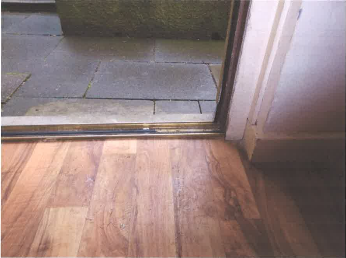
Ground floor Front door threshold rubber strip damaged – to be replaced.
