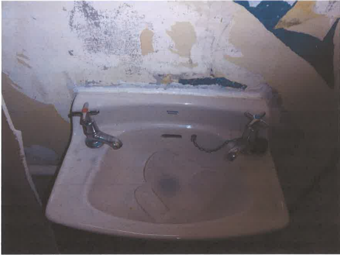
Ground floor toilet; Wash hand basin fixed to wall; To finish
