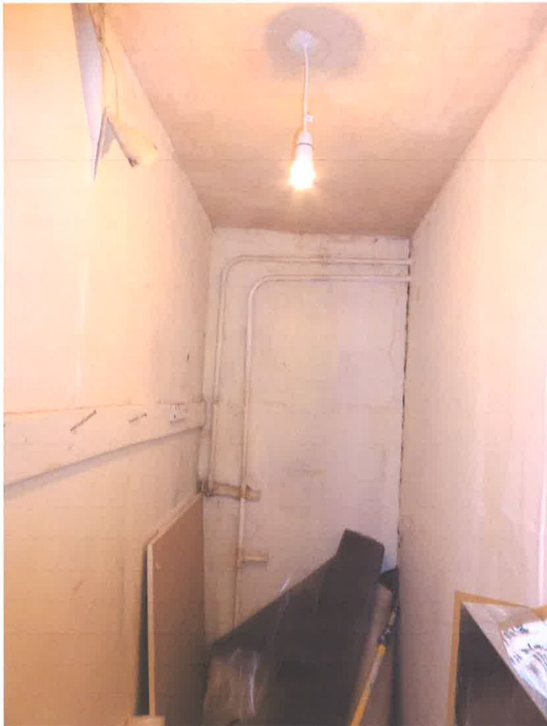
Ground floor cupboard; Ceiling repaired and plastered. End wall remains damp.
