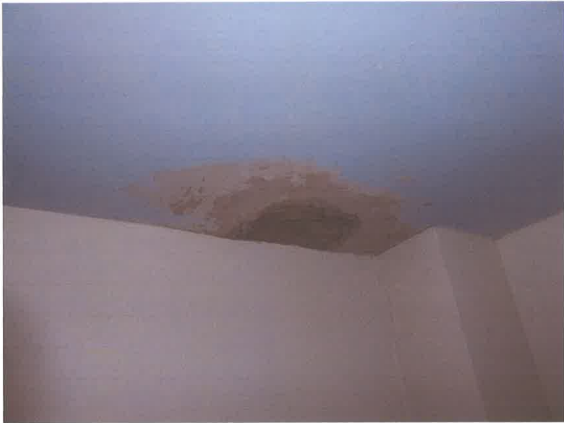
Top Floor – North bedroom ceiling repair following leak above repaired but not finished
