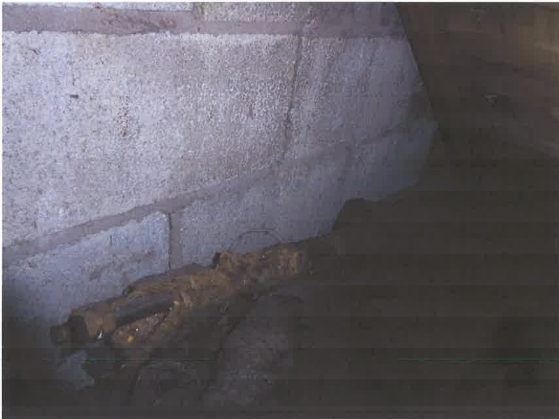
Loft – cut off cold water pipes also above area of damaged ceiling. No leaks evident.
