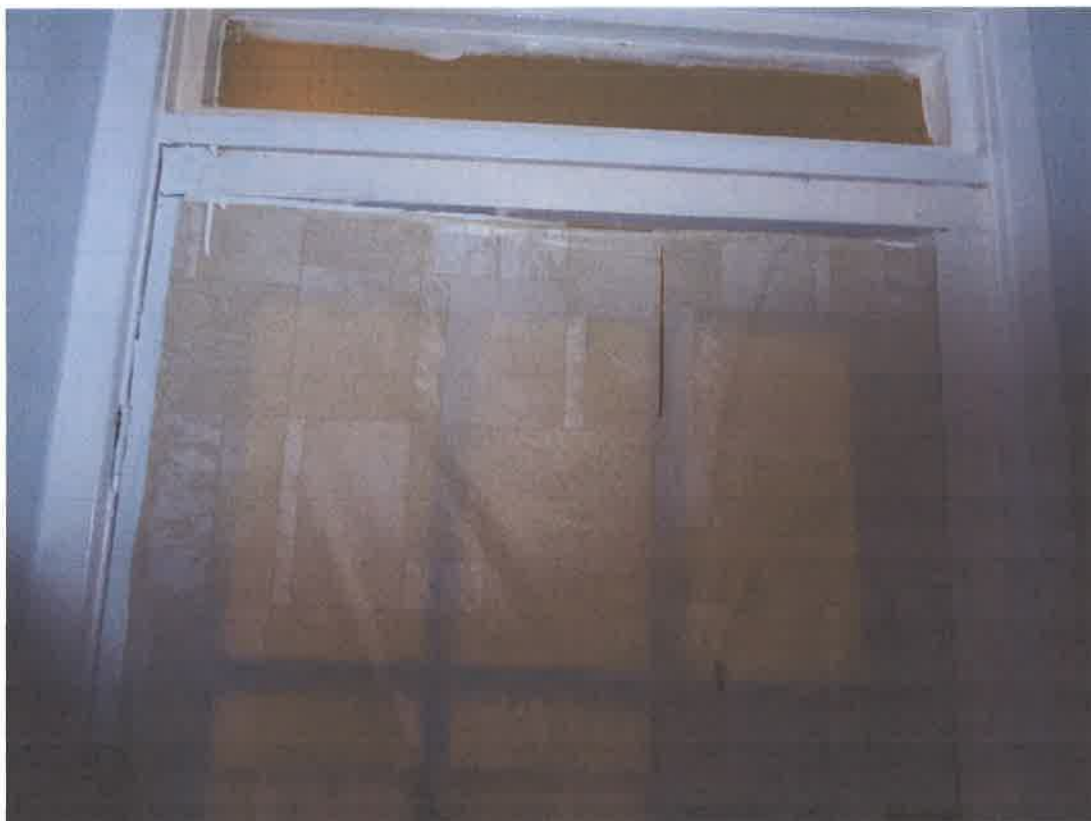
Middle Floor bedroom door; Poor fitting former 15pane glazed door inappropriate for bedroom – to be replaced.
