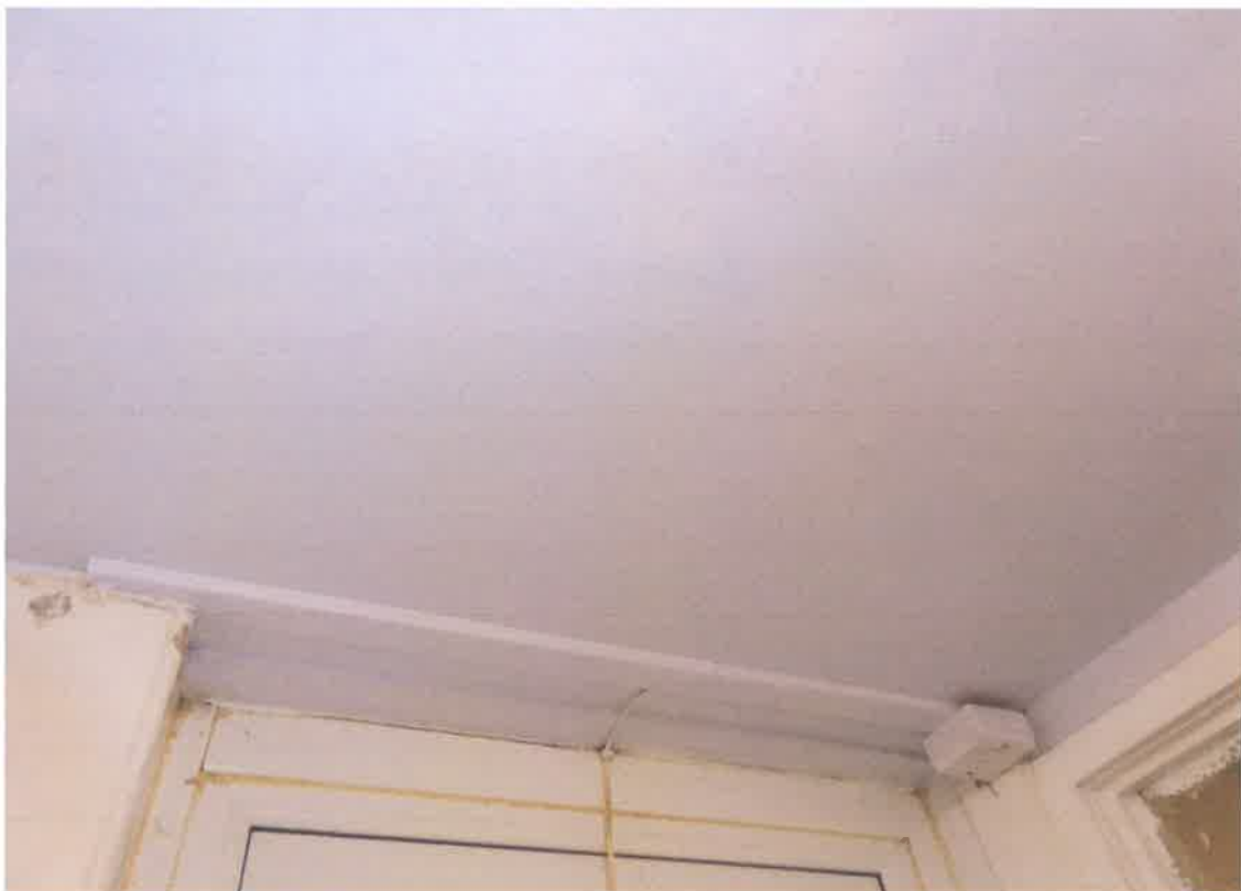
Ceiling freshly painted. Expelair cut out switch should not be within bathroom
