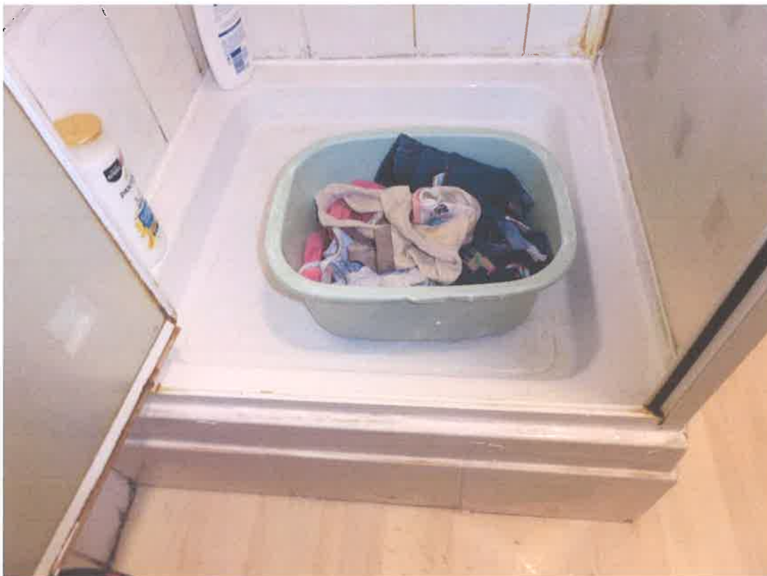
Shower tray – external view. High step up into shower and damaged flooring (damp) in front of door
