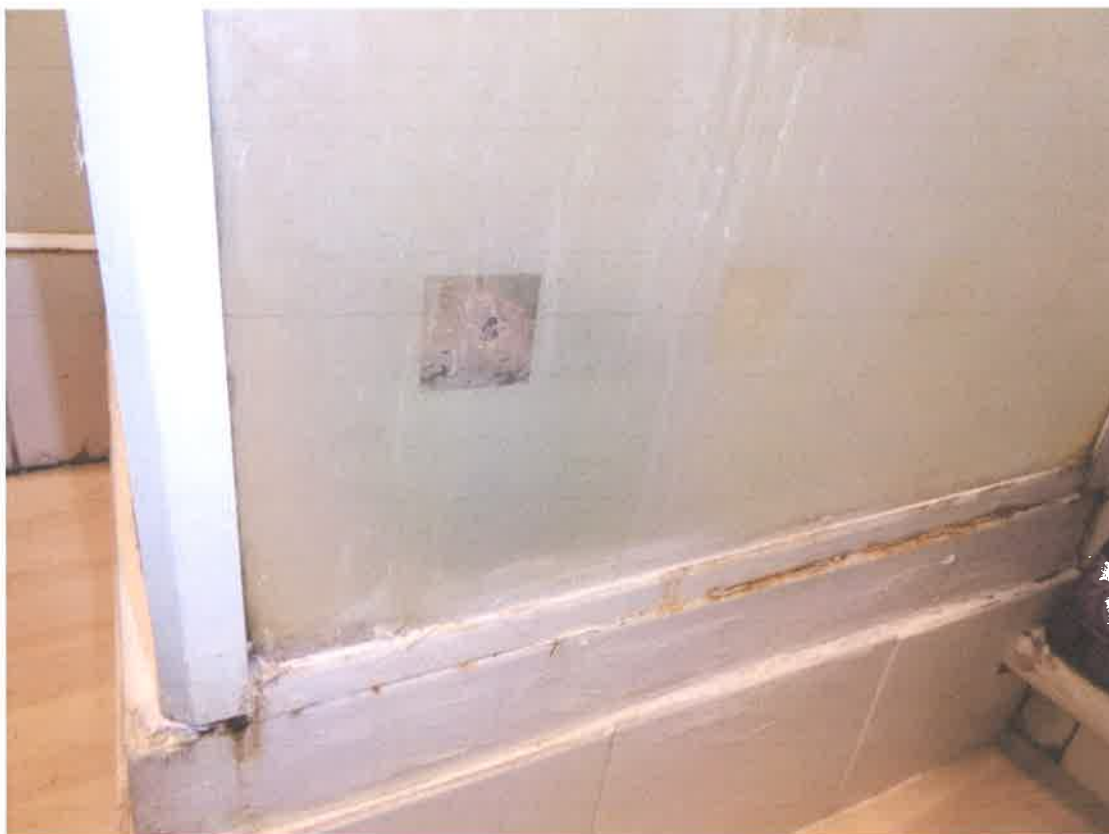
Shower tray side. Resealed with silicone but showing signs of age (rusting frame)
