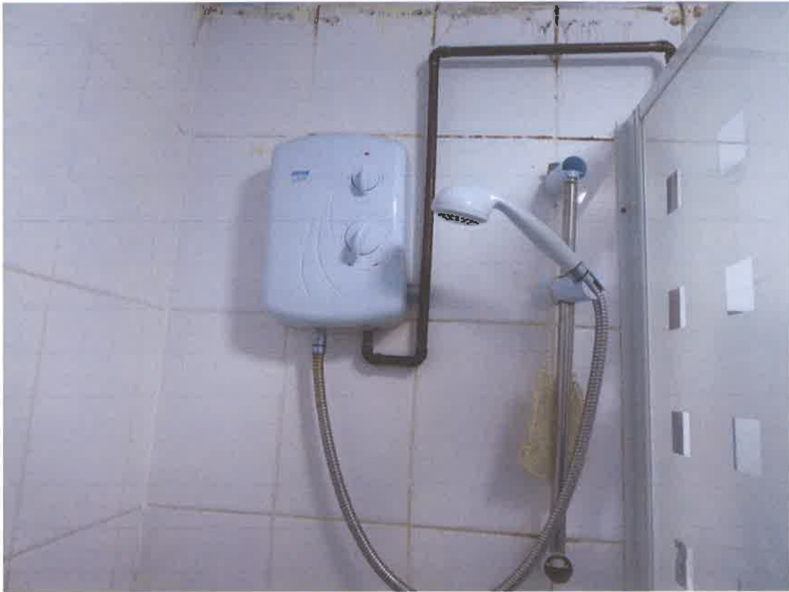
Middle Floor shower working properly but shower head guide rail loose at top (not properly fixed)
