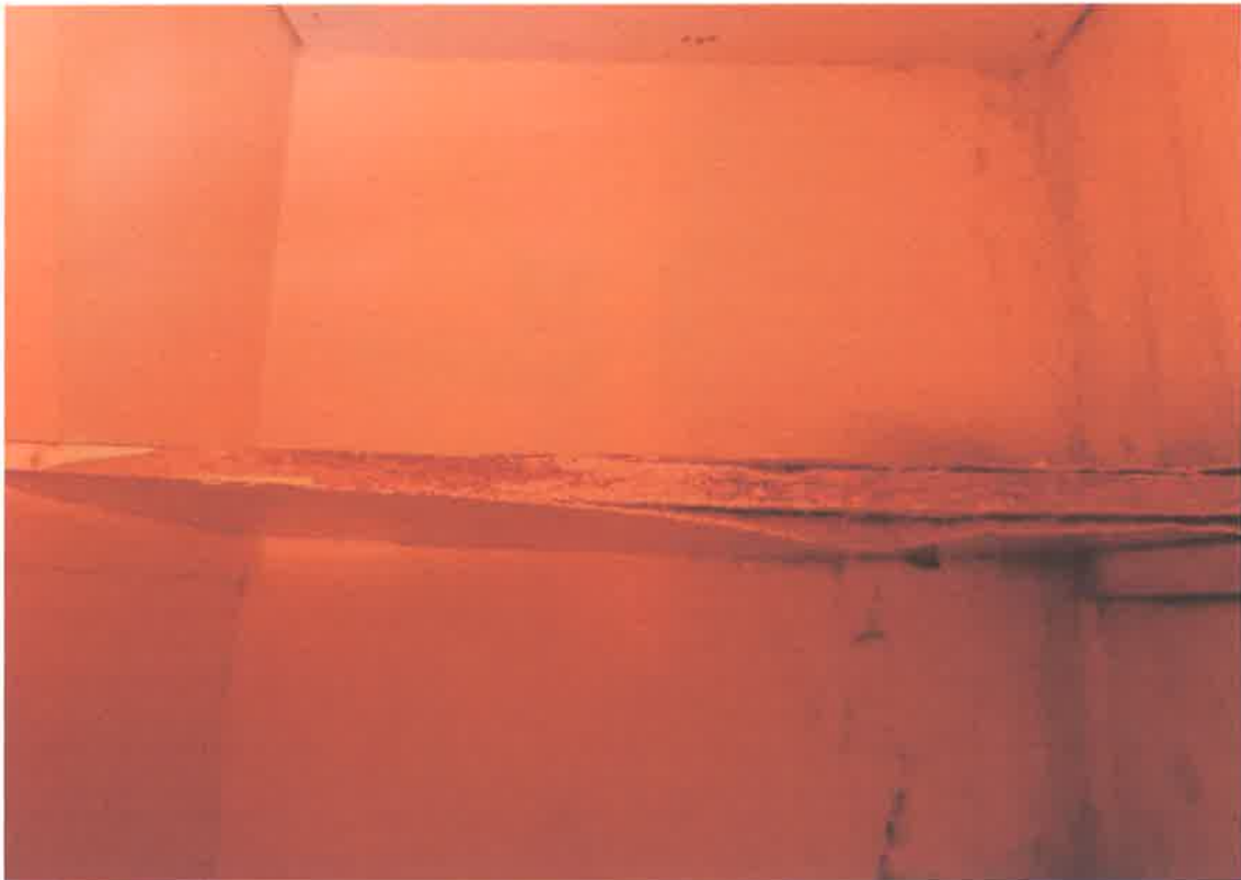
Ground floor kitchen cupboard; end wall remains damp in upper half. Shelving to replace.
