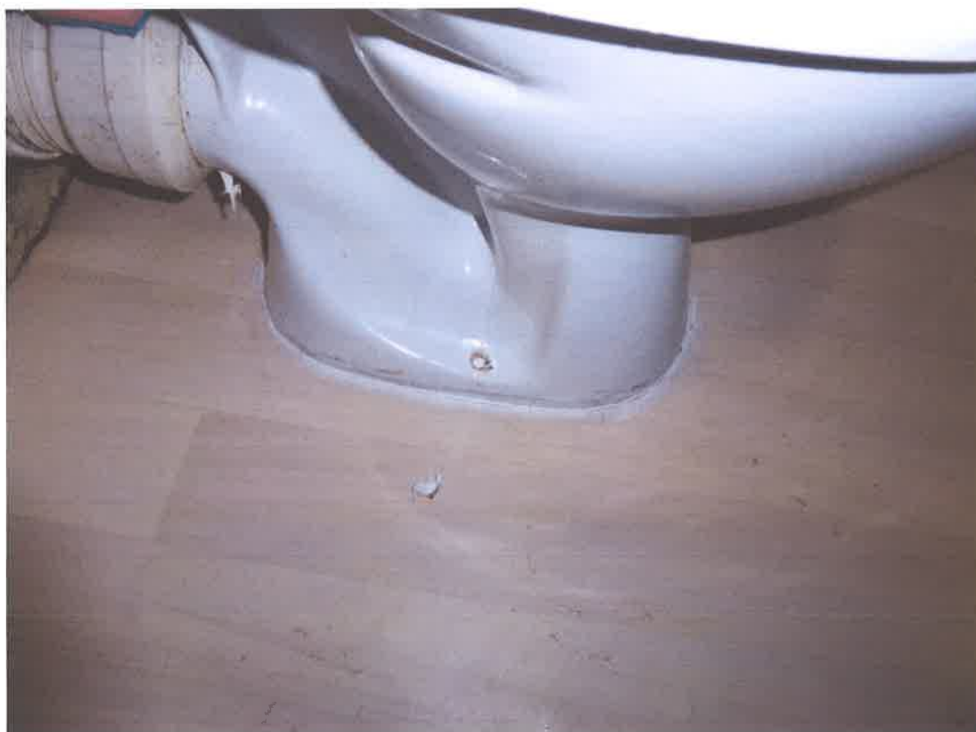
Middle Floor Shower room WC – not screwed down. WC rocks and cistern not fixed to wall
