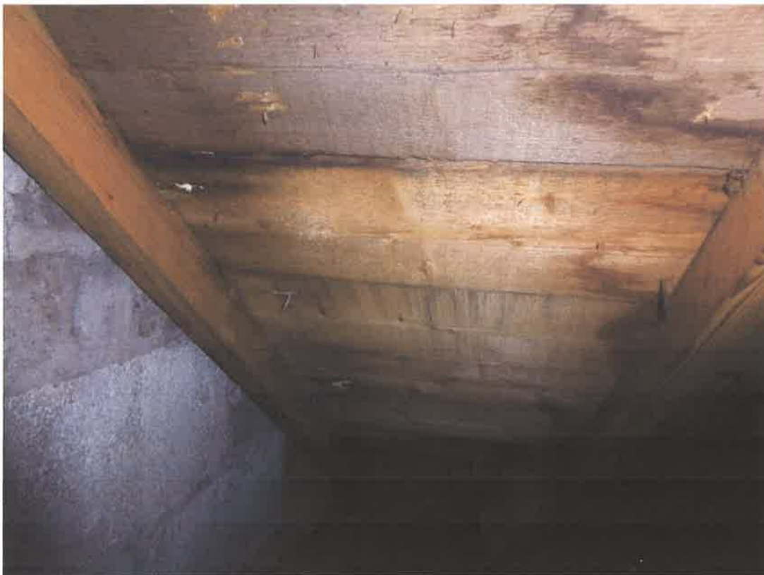
Loft - Close up of roof sarking – discoloured area showing evidence of former leak.
