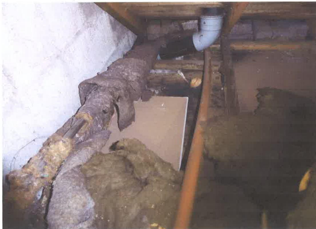
Loft gable wall; Ceiling to North bedroom plasterboard repair patch. Evidence of damp from roof sarking but dry now
