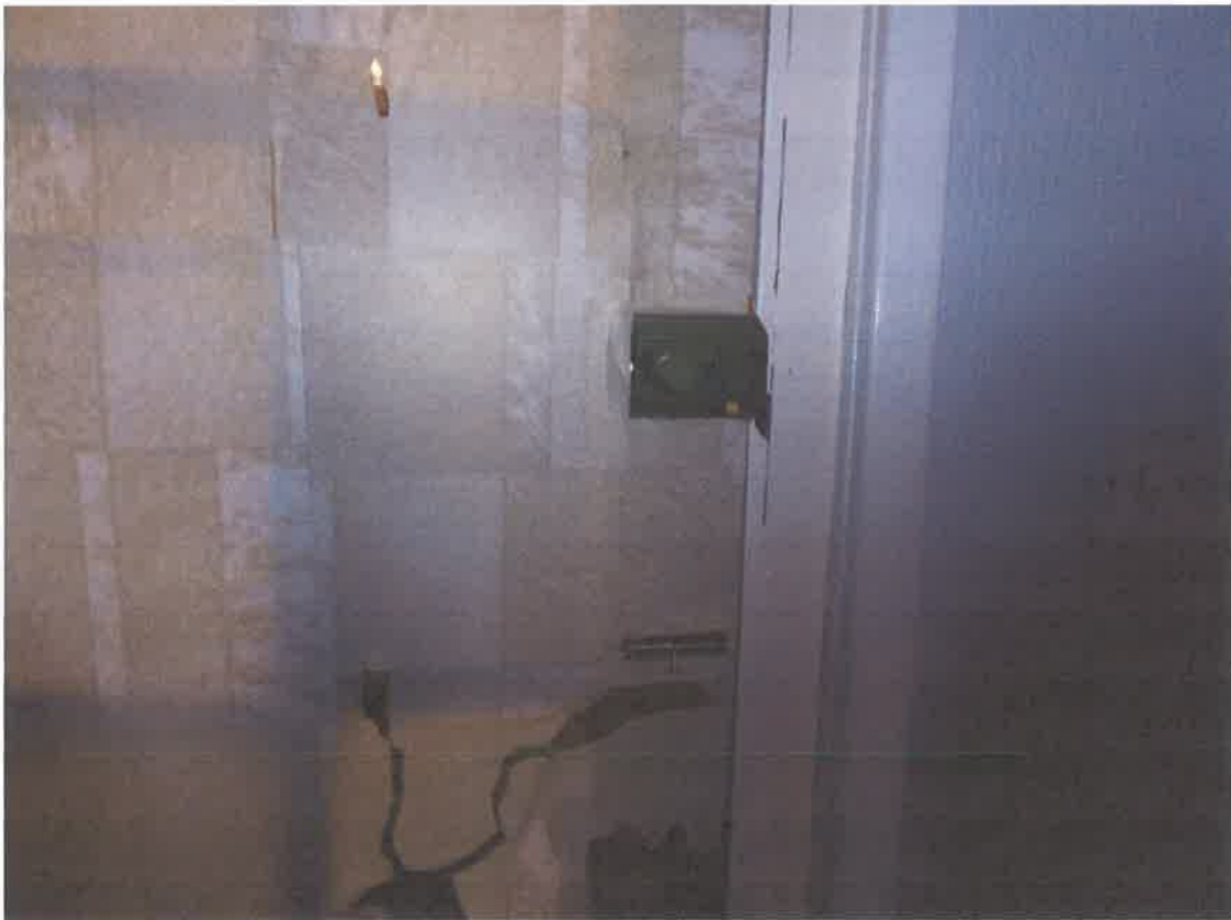
Middle floor door yale lock with no keeper. Note door papered over by tenant
