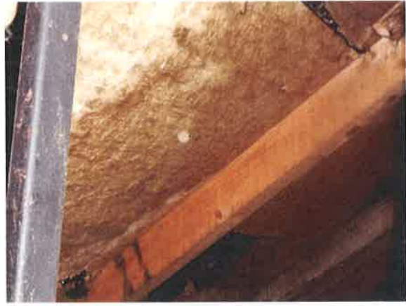
10:- Sarking & insulation in attic
