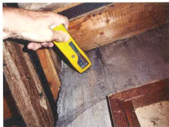
13:- Staining chimney plaster – dry
