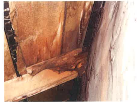
12:- Staining at sarking – dry
