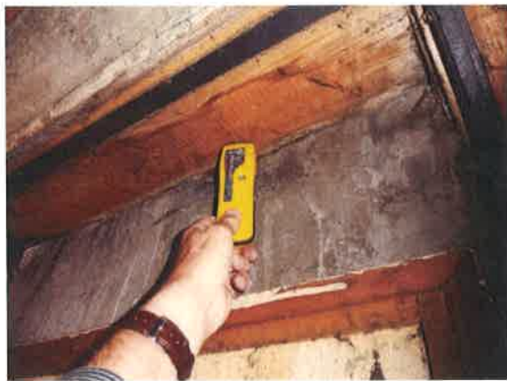
11:- Staining by chimney - dry
