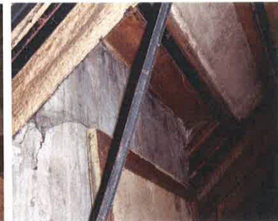
14:- Staining at sarking - dry
