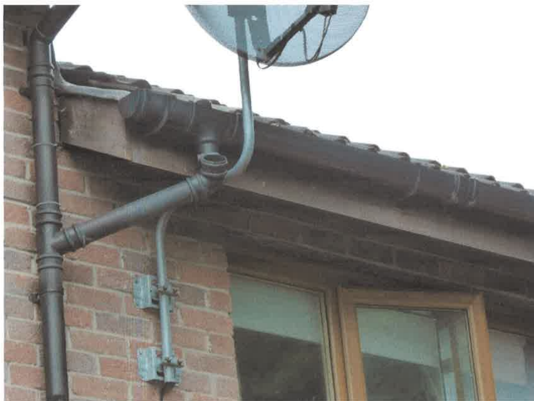
Front elevation. Downpipe unattached to gutter
