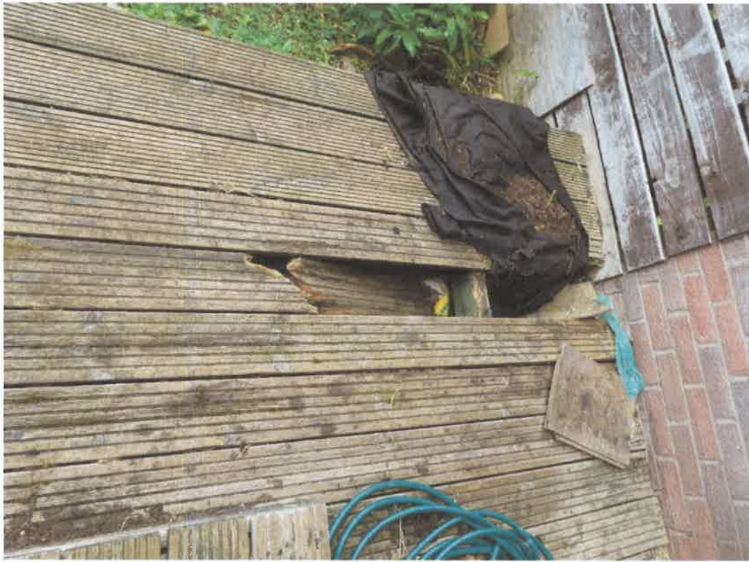
Decking to rear door / garden. Rotten and unsafe
