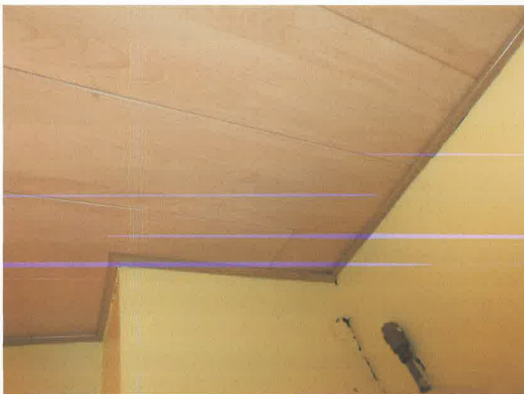
Kitchen ceiling below bath waste. Possible damage from ingress of water – see distorted panel.
