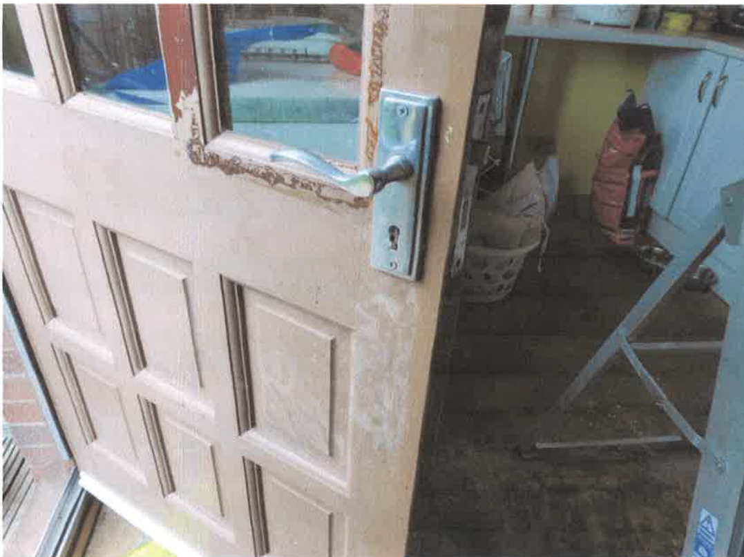
Rear door – lock not working and screws missing from lock coverplate
