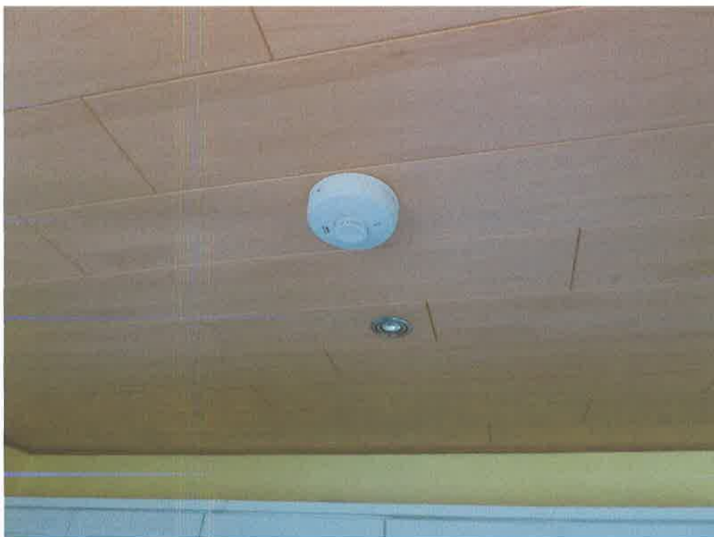
Heat detector in kitchen – fitted but not tested. Not a combined CO alarm
