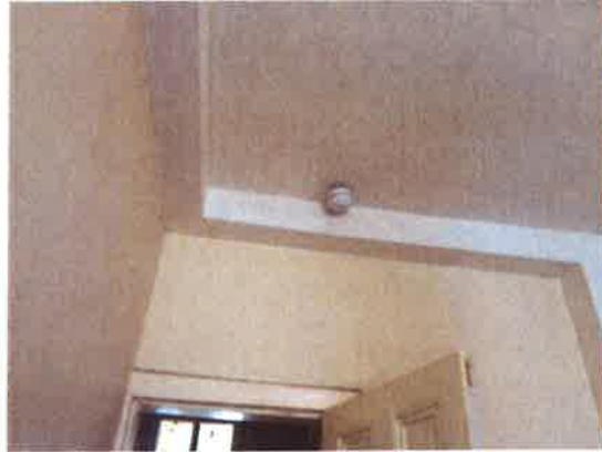
Hardwired Smoke detector fitted
