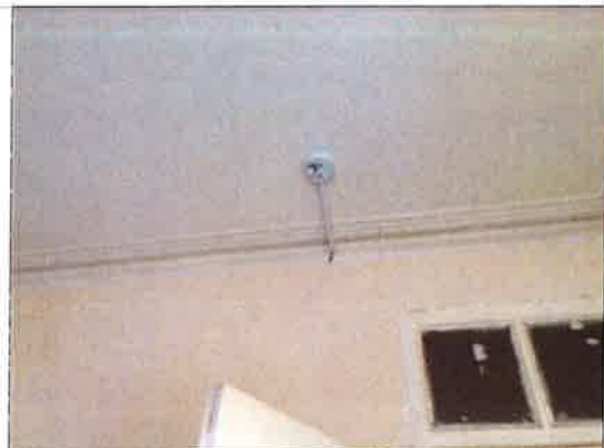
Hardwired Smoke detector base fitted No Smoke detector attached
