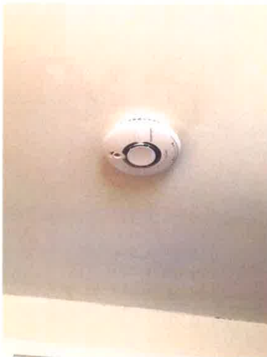
Photograph 5: Upper hallway – smoke detector
