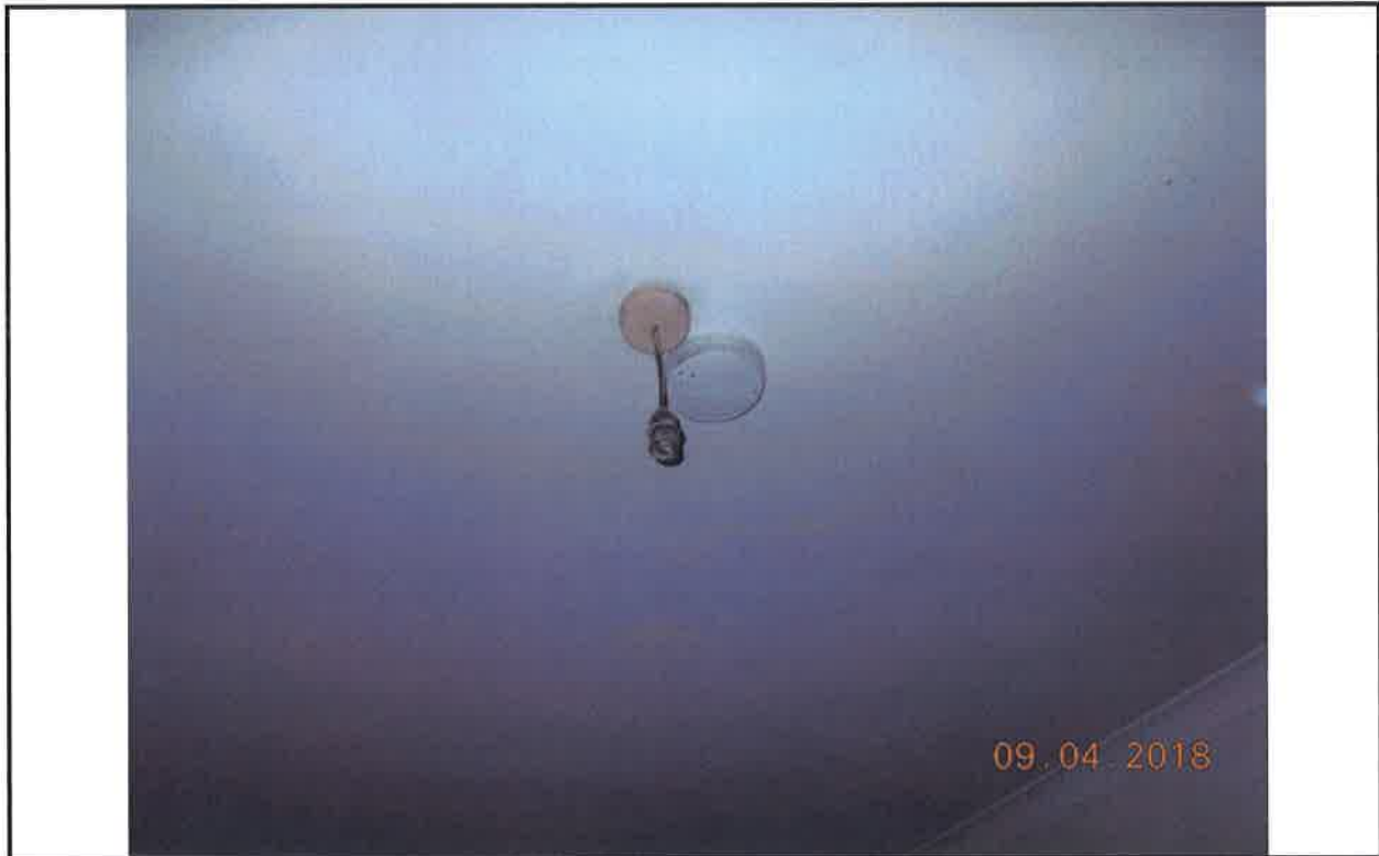
3. Defective light fitting in Bedsitting Room
