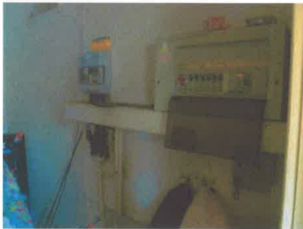
18. Electric meter and consumer unit
