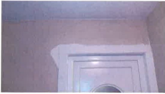
Photo 6 - Repair to flat entrance door
