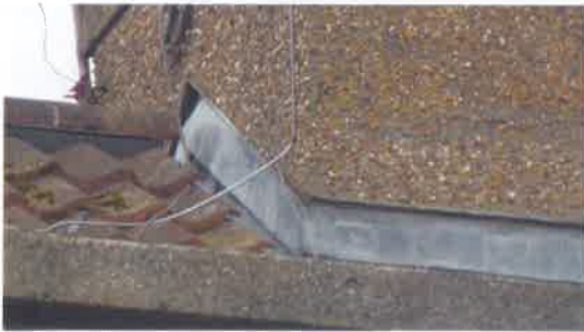
Photo 10 -Lead flashing detail on C/Head
