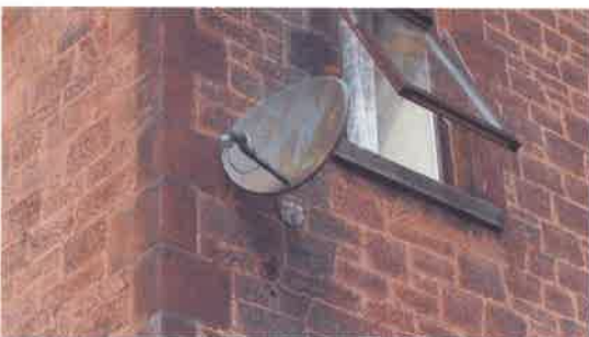
Photo 6 – Corresponding wall section
