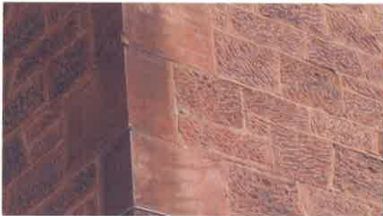
Photo 4 – Corresponding wall section
