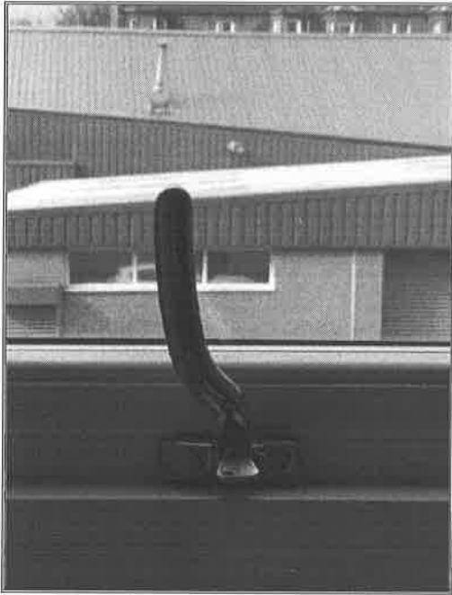
Photographs 7 and 8: replacement handles to kitchen windows
