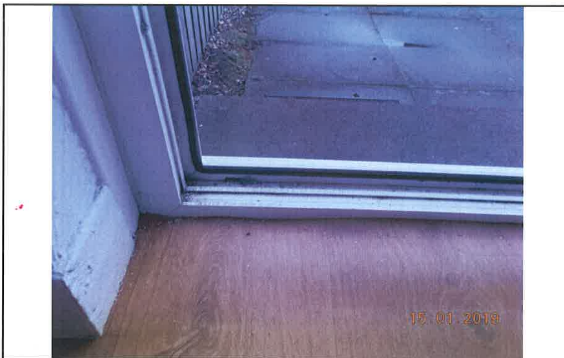
7. Cill of rear door with score marks at opening edge
