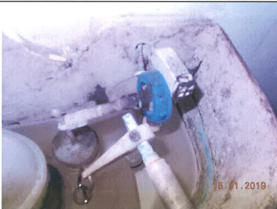
9. Loose fixing screw to cistern
