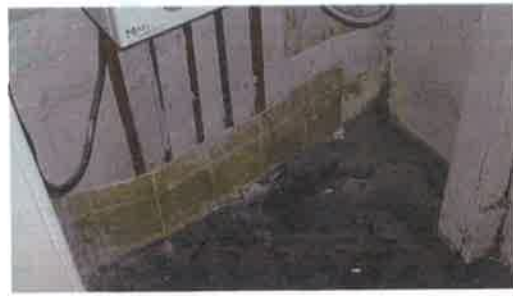
Photo 3 – Rodent access in kitchen
