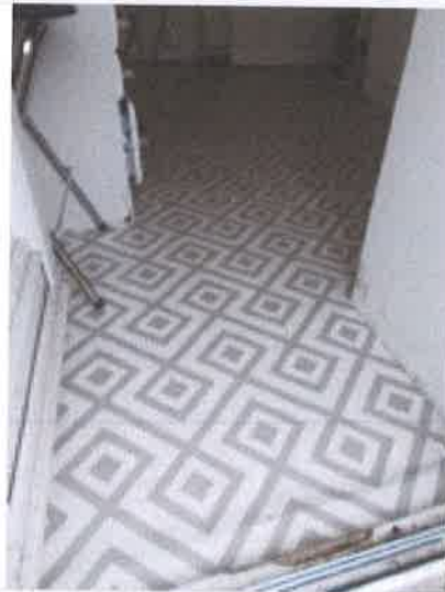
Kitchen - tiles removed/new vinyl floor covering
