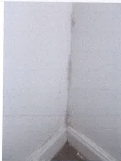
Bathroom - black spot mould in corner
