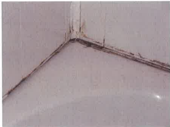
7. Substantial gap at "wet wall" & bath
