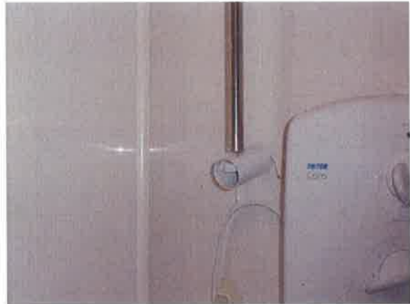
5. Broken showerhead rail support
