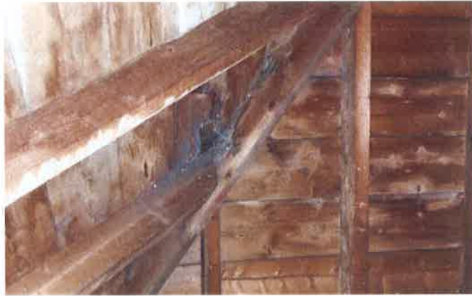
16. Hole in timber sarking in attic exposing bitumin underfelt below external roof tiles.
