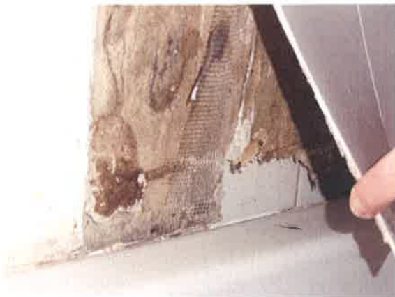
6. Poorly secured "wet wall" at shower
