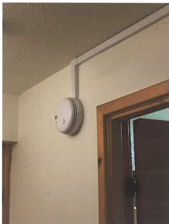
Photograph 7: Hall: smoke detector
