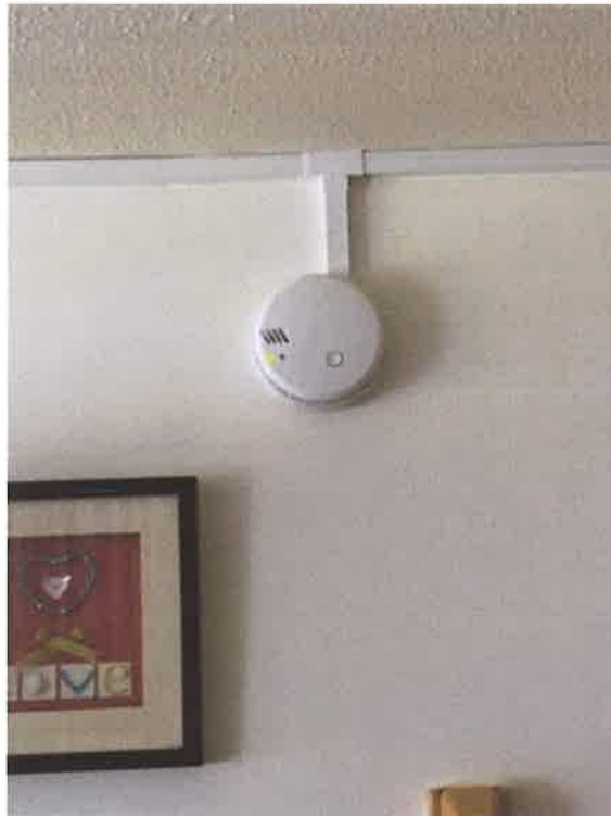
Photograph 7: Hall: smoke detector
