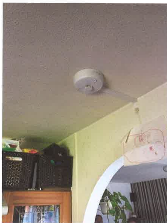
Photograph 5: Kitchen: heat detector
