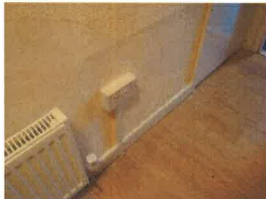
HALL-LOOSE WIRING TIDIED UP
