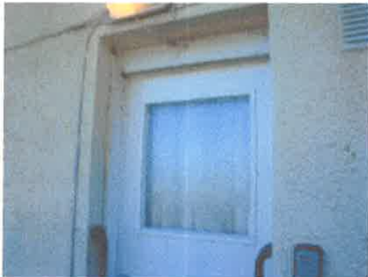
KIT DOOR-SILICONE SEALS POOR
