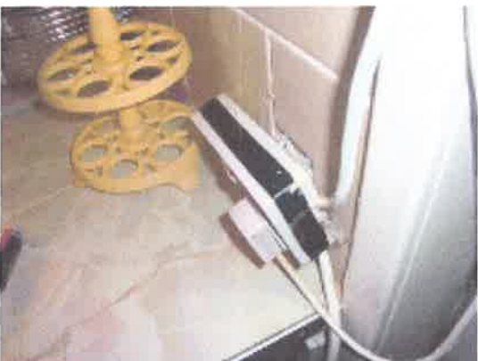
KIT –DOUBLE GANG SOCKET LOOSE
