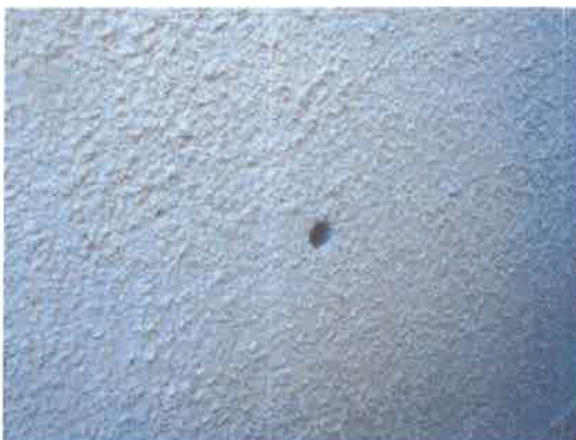
HOLE IN RH GABLE WALL
