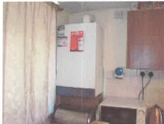
KITCHEN - CH BOILER- NO CO MONITOR
