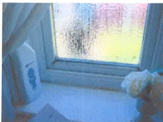
WC APT-INTERNAL CONDENSATION
