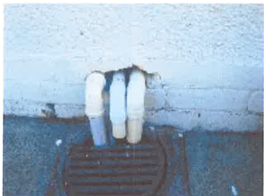
PIPES/GAPS IN FRONT ELEVATION
