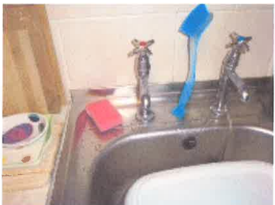
KIT SINK – LEAKING TAP
