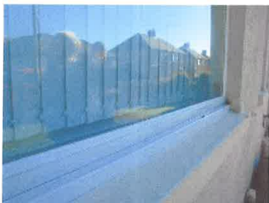
KIT WINDOW-BROKEN SEAL
