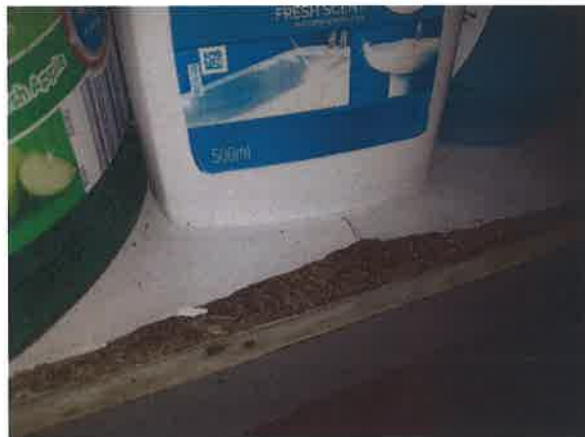
15 Base unit water damaged in Kitchen.
