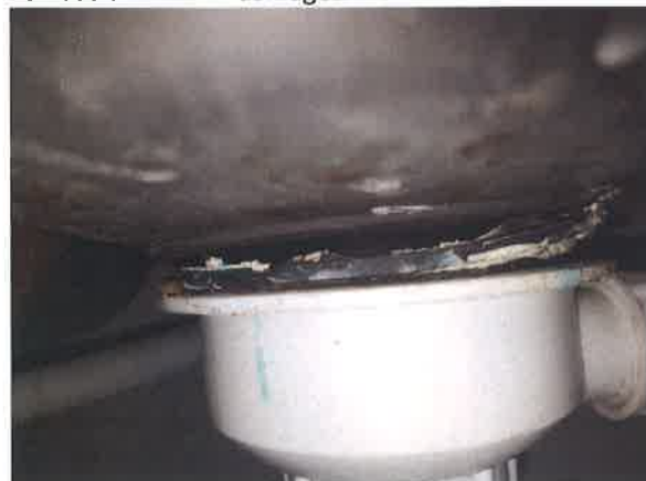
17 Unconnected waste at kitchen sink.
