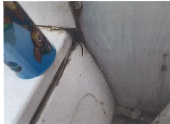
6 Damaged bath panel.
