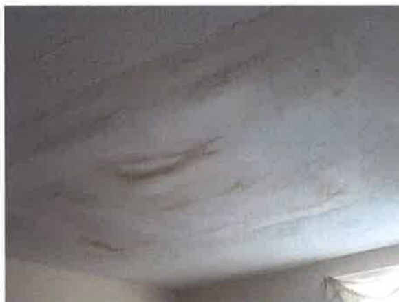
8 Water damage to ceiling.
