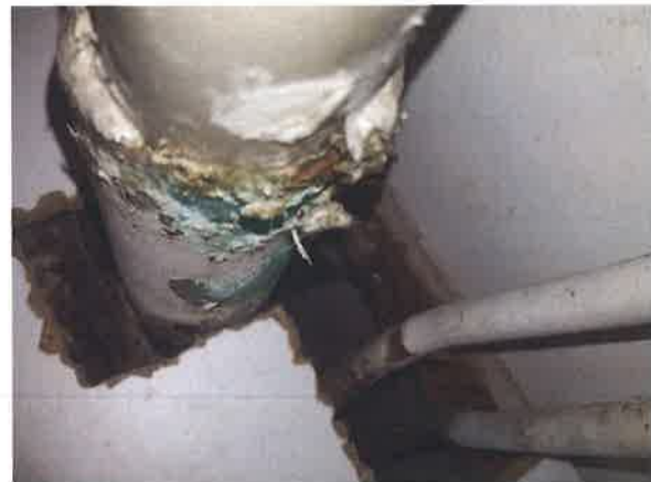
16 Poor joint to pipework and leaking.
