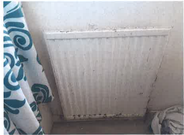
4 Corrosion to radiator in bathroom.
