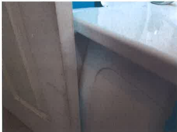
5 Poor fitting of bath panel.
