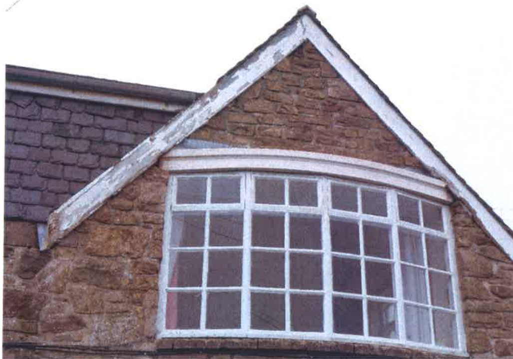
South West gable / flat roof abutment. Slate missing at junction of flat roof/ barge board
