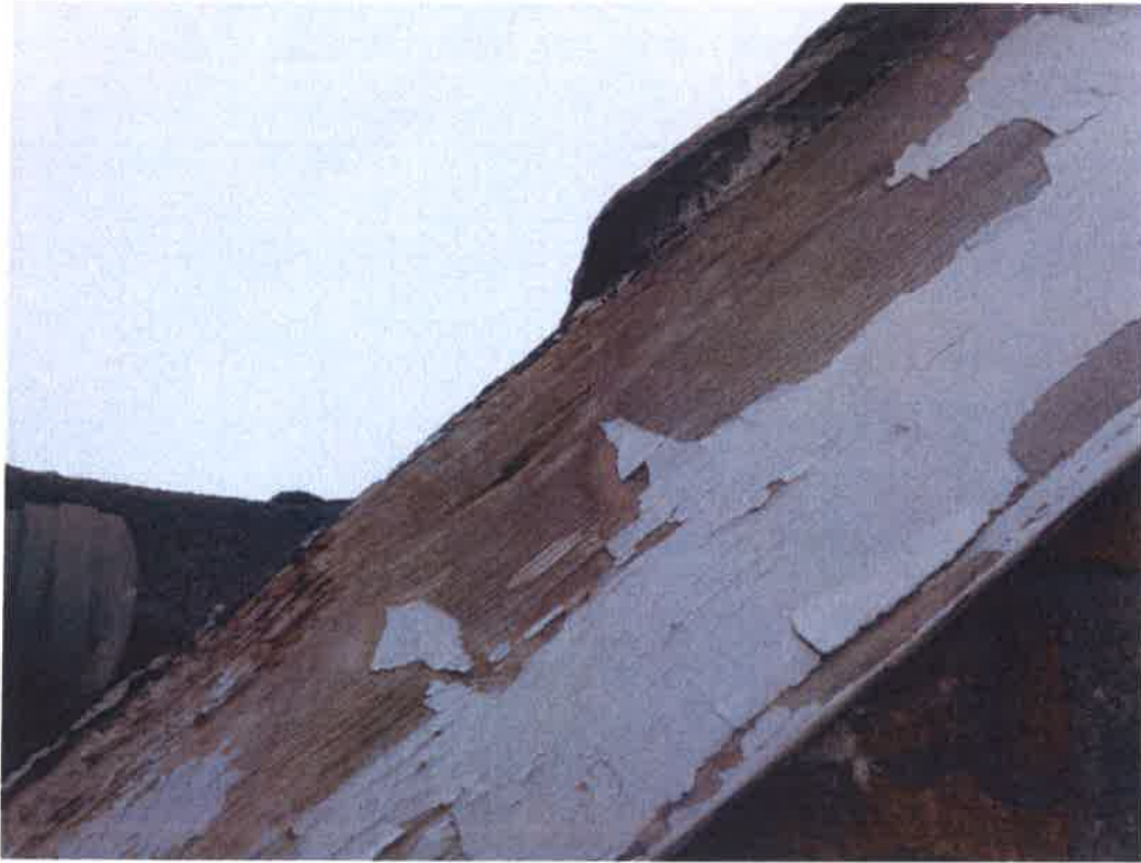
Close up of missing slate above and decaying barge board
