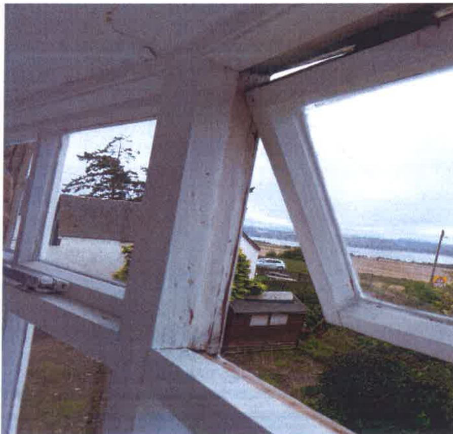
Top opening section of NE bedroom window – no draught-proofing
