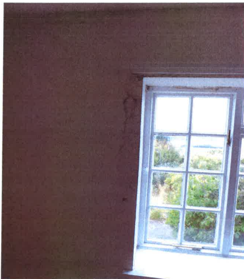
Damp to head and side of window in central bedroom beneath flat roof
