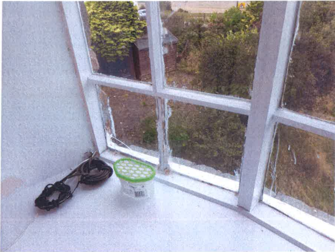
North East 1 st floor bedroom. Damaged astragal and cracked bottom pane
