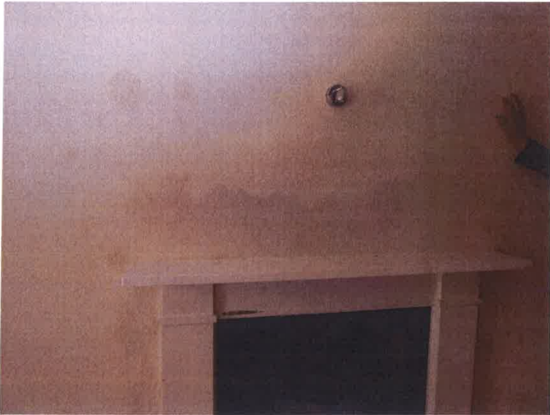
Damp wall above and to side of fireplace in ground floor South West gable bedroom
