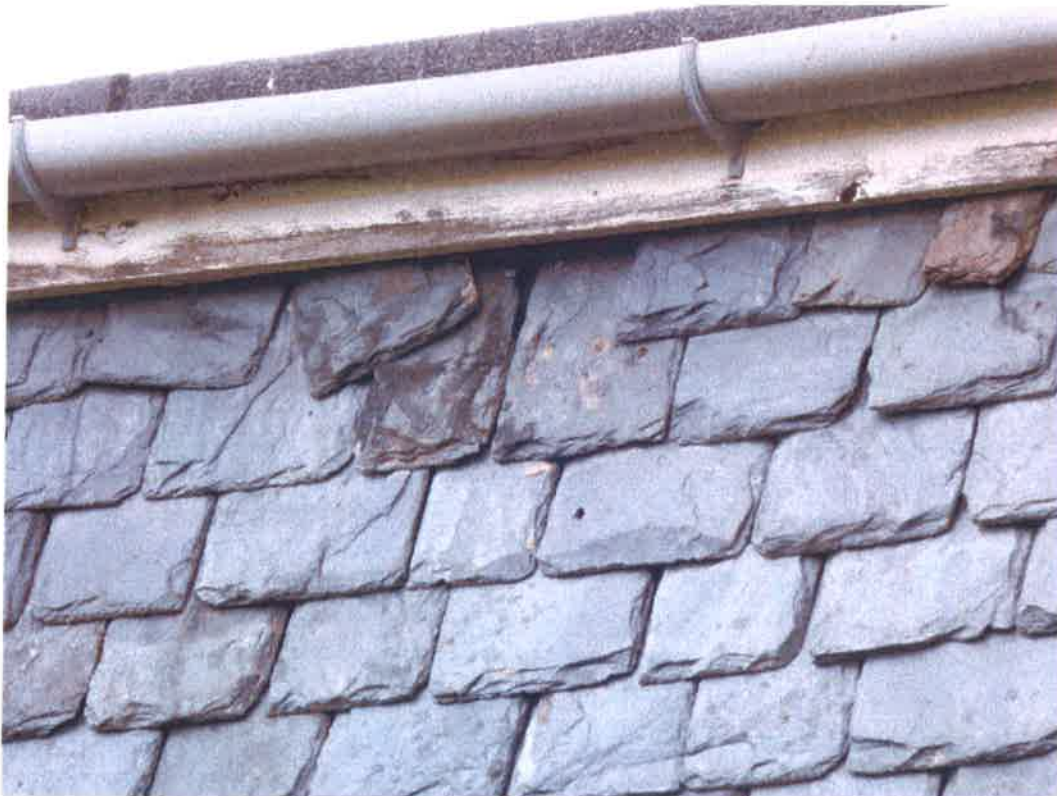
Loose and missing slates from mansard section below flat roof
