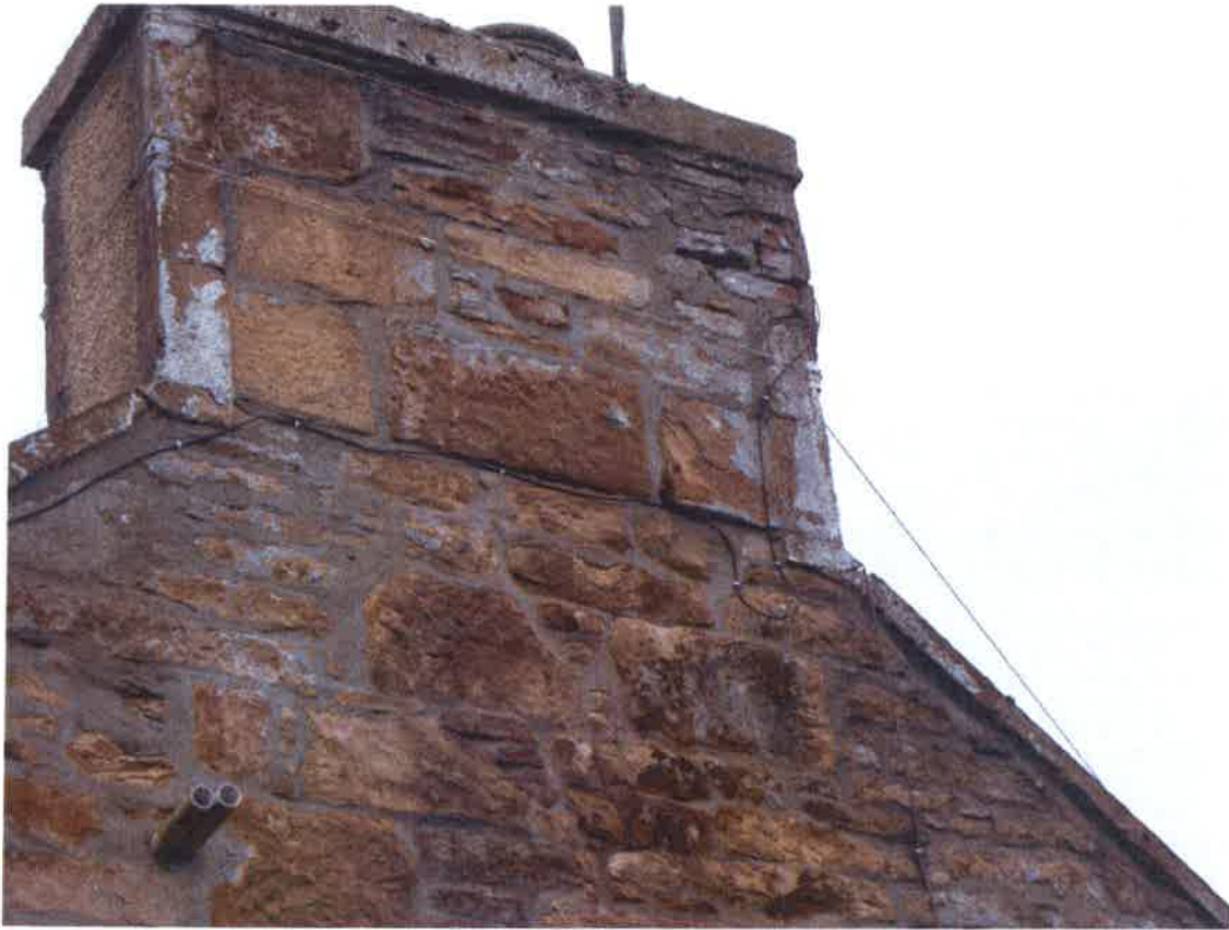
Damaged / missing pointing from chimney on North East gable (middle right of stack)
