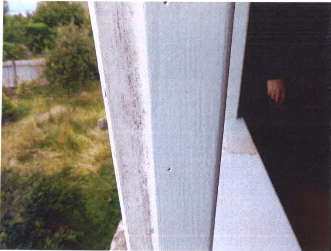
Opening section of window in central bedroom (below flat roof) – no draught-proofing
