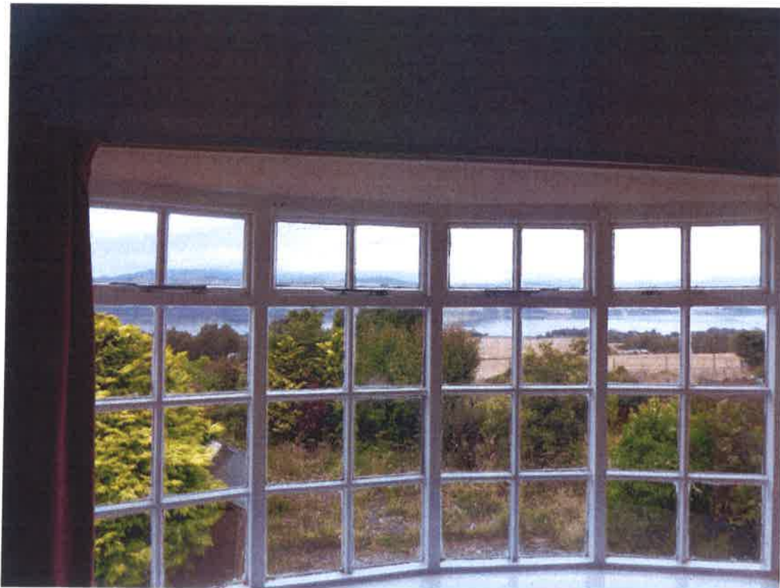
Master bedroom (SW Gable) window in rear elevation showing opening sections
