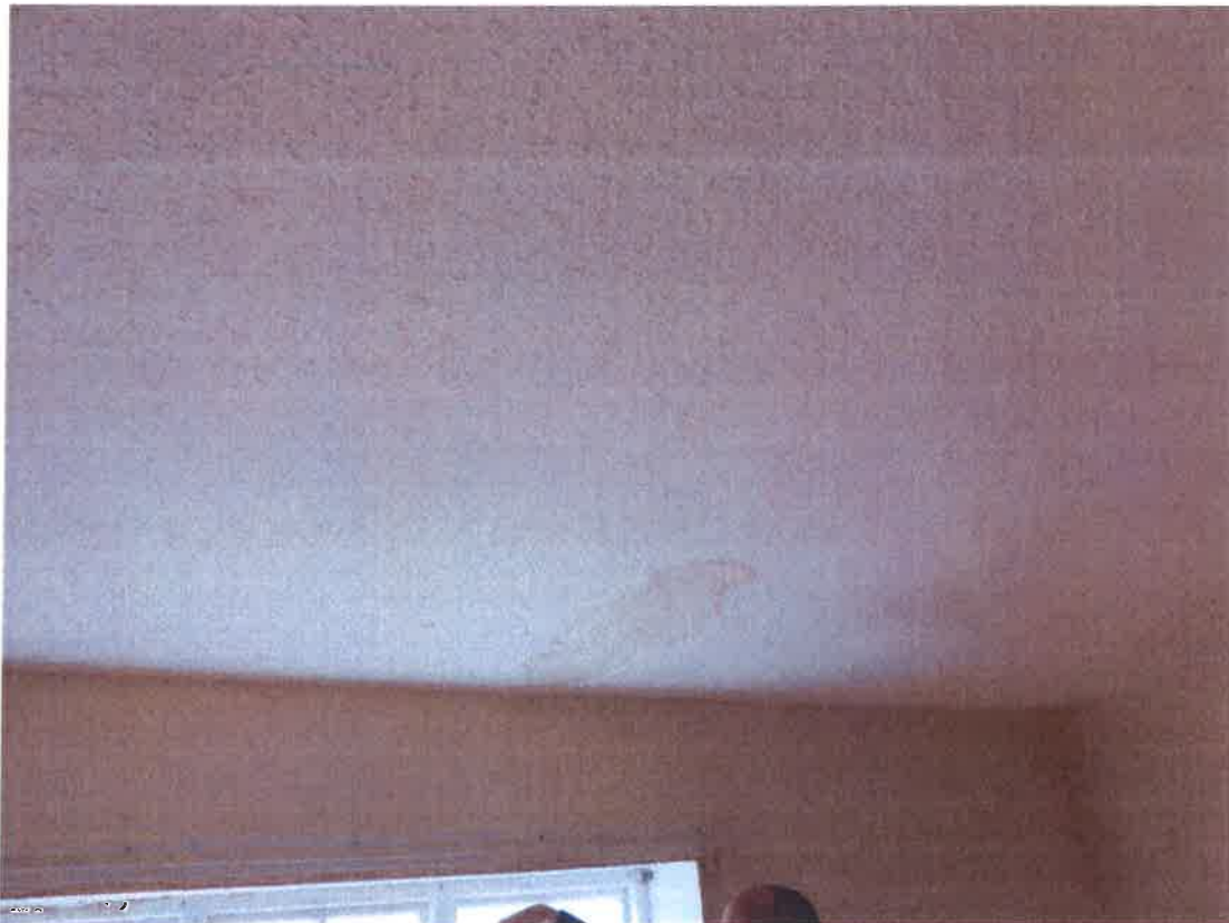
Damp ceiling to central bedroom under flat roof
