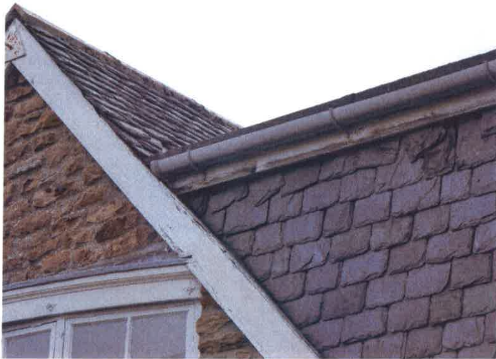
North East gable / flat roof abutment showing slate missing above flat roof
