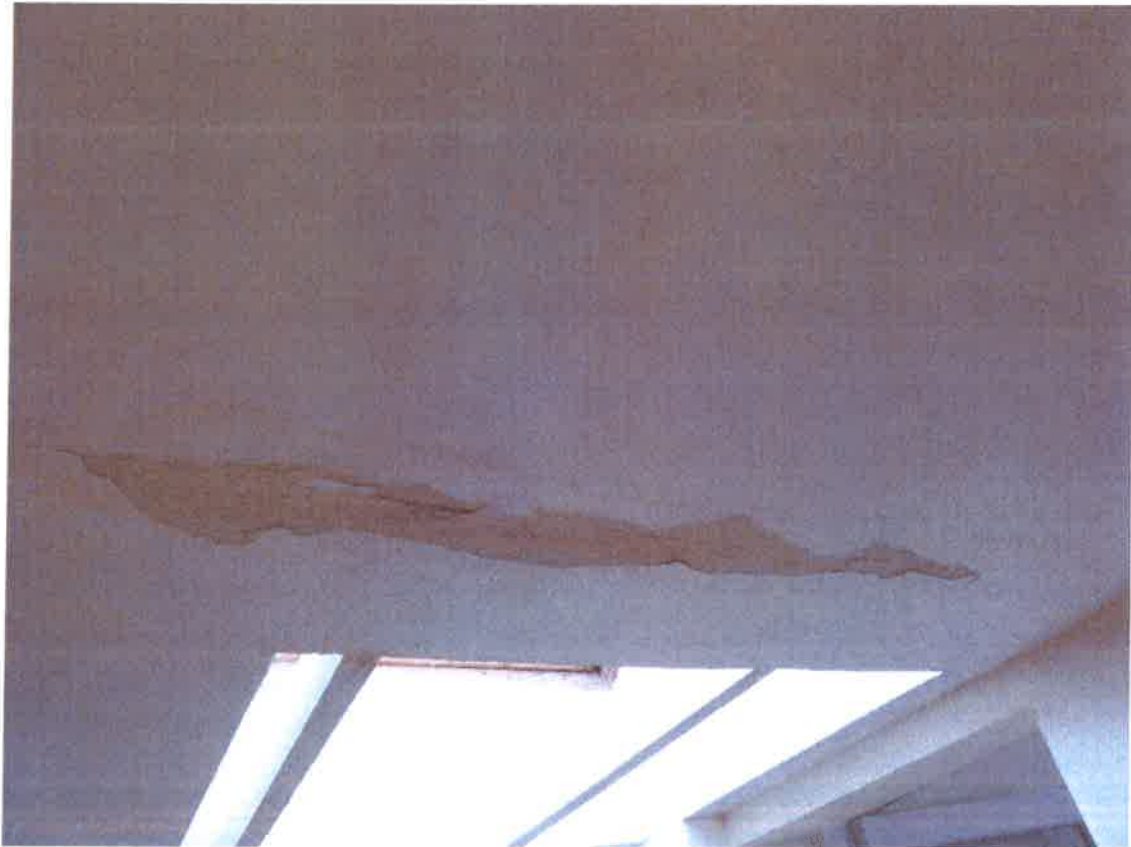
Damp patch in ceiling of single storey lounge extension (below slated roof).
