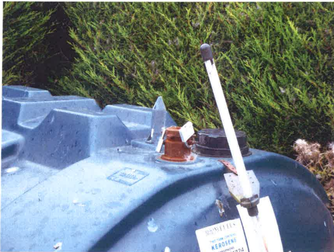
Oil tank with locks on filler cap.
