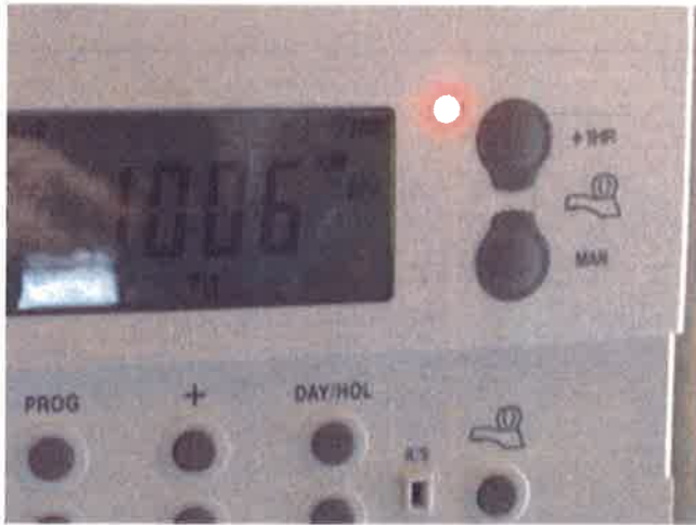
5. Close up of boiler control panel in kitchen including hot water booster switch
