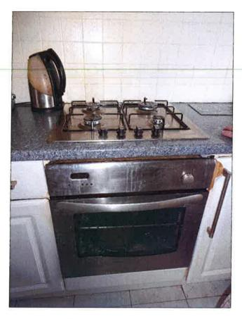
Gas burners on hob have been fixed by landlord all 4 tested at inspection, however the tenant advised gas oven was disconnected from gas supply by gas engineer.
