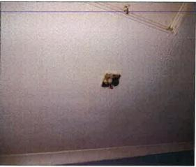
Smoke detectors in hall and first floor landing are battery operated and at time of inspection not in operation. The kitchen had no means of detecting fire.
