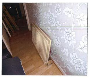
Radiator in the second bedroom is hanging off wall. Radiator in main bedroom is off wall and sitting on floor still connected to the heating system.
