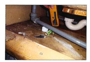
Waste pipe under sink is leaking
