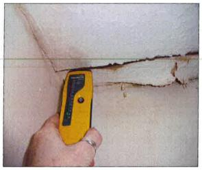
Dampness in kitchen - moisture reading taken during inspection showed normal reading however historic water ingress was noted. Areas of mould appears to be due to condensation as no trickle ventilation or mechanical ventilation was present.
