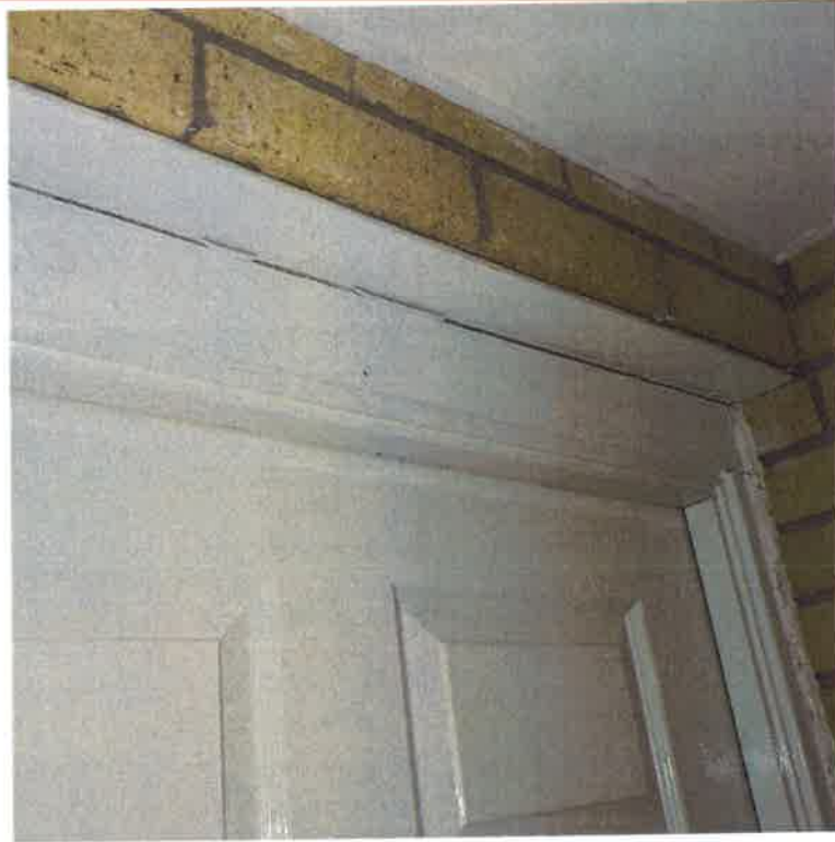
2 The split frame at the door head above the front entrance door
