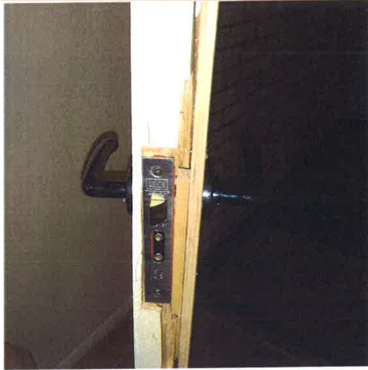
4 The split and patched leading edge of the front entrance door at the lock/handles
